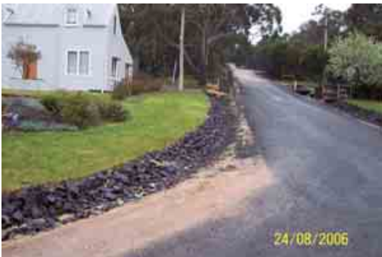
Figure 22 Rocks Lining of Drains
