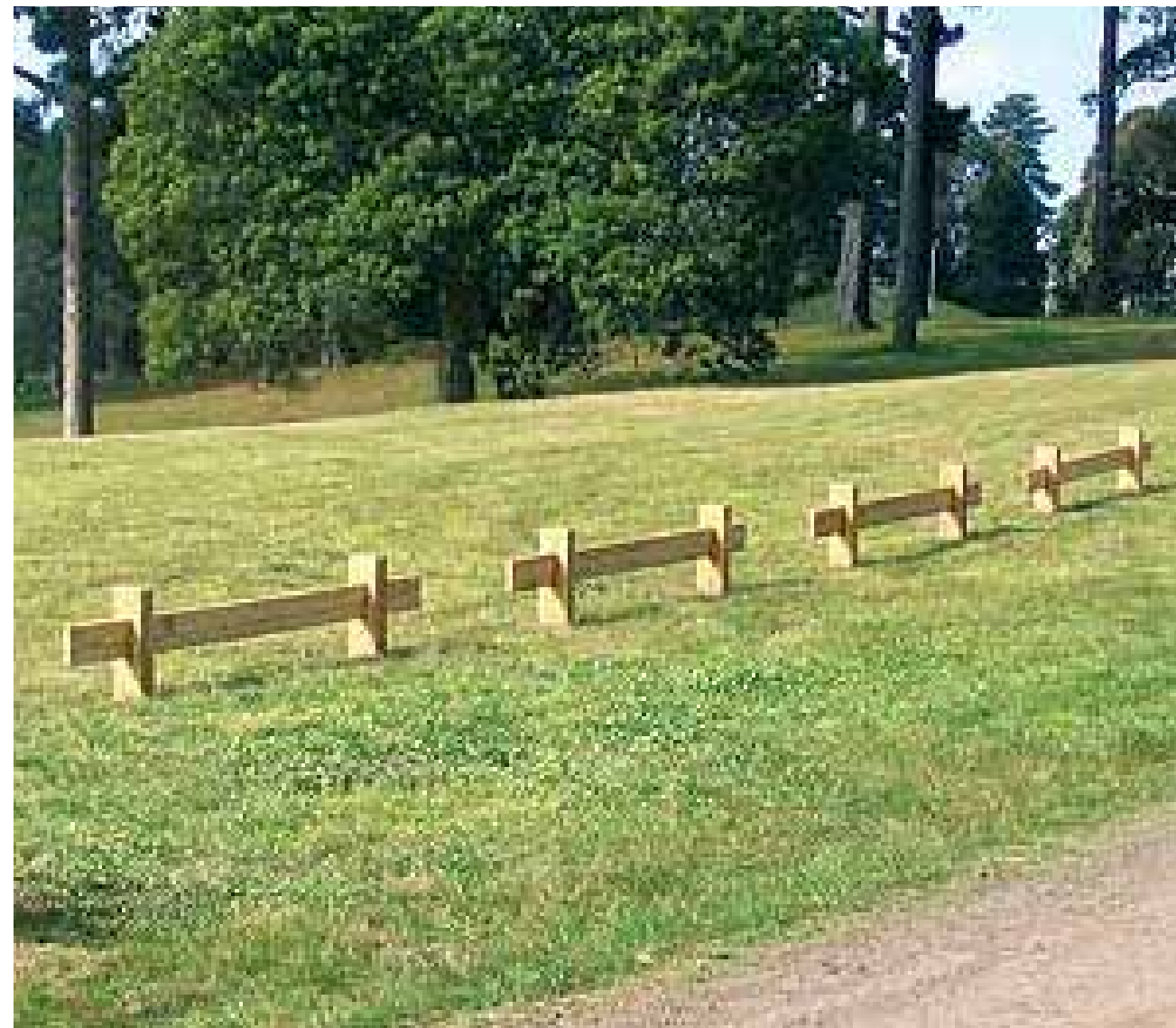
TIMBER POST & RAIL FENCE To be provided between reserve and existing road reserve.
