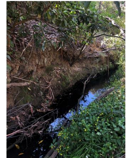
Photo 4 – Below informal timber crossing of Deep Creek (looking downstream). Waterway is incised with evidence of bank undercutting. Right bank vegetation becomes more cleared allowing introduced grasses to enter the riparian zone.
