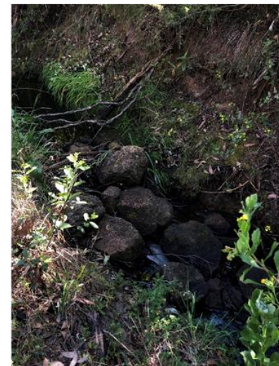
Photo 5 – Informal rock structure in Deep Creek. Rocks have been placed to reduce bed deepening with noticeable effect on water levels upstream and downstream.
