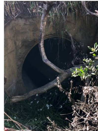
Photo 3 – Upstream end of culvert at Deep Creek crossing. Pipe diameter is approx. 1.5m.
