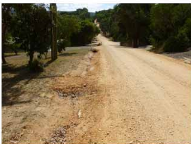
Looking north towards Kurrjong Avenue and Aireys Street.
