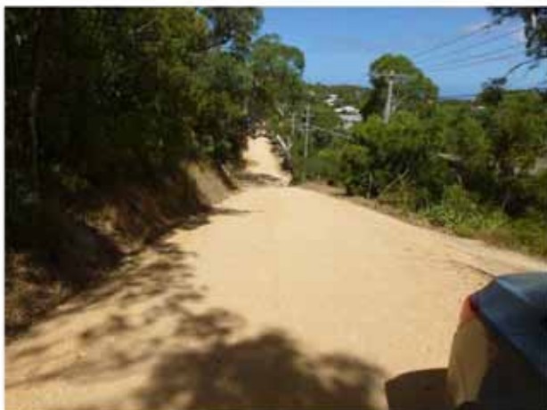
Looking south to Aireys Street intersection.
