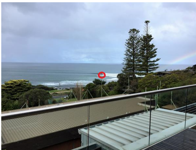
Photo 3 – Circle indicates the 9.6 metre wall height which impacts on views of breaking waves. Source: Planning Officer
