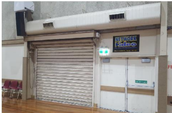
Figure 5: Roller door and emergency exit on south-west wall
