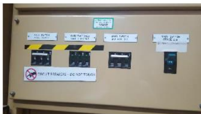
Figure 2: Main switches
