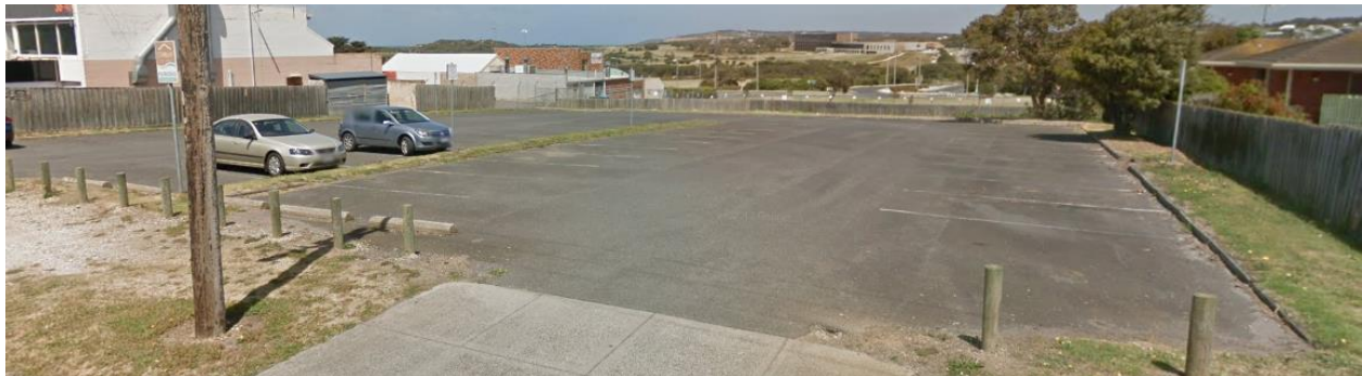
Photo 3 – Car park on Rudd Avenue. Source: Google street view
