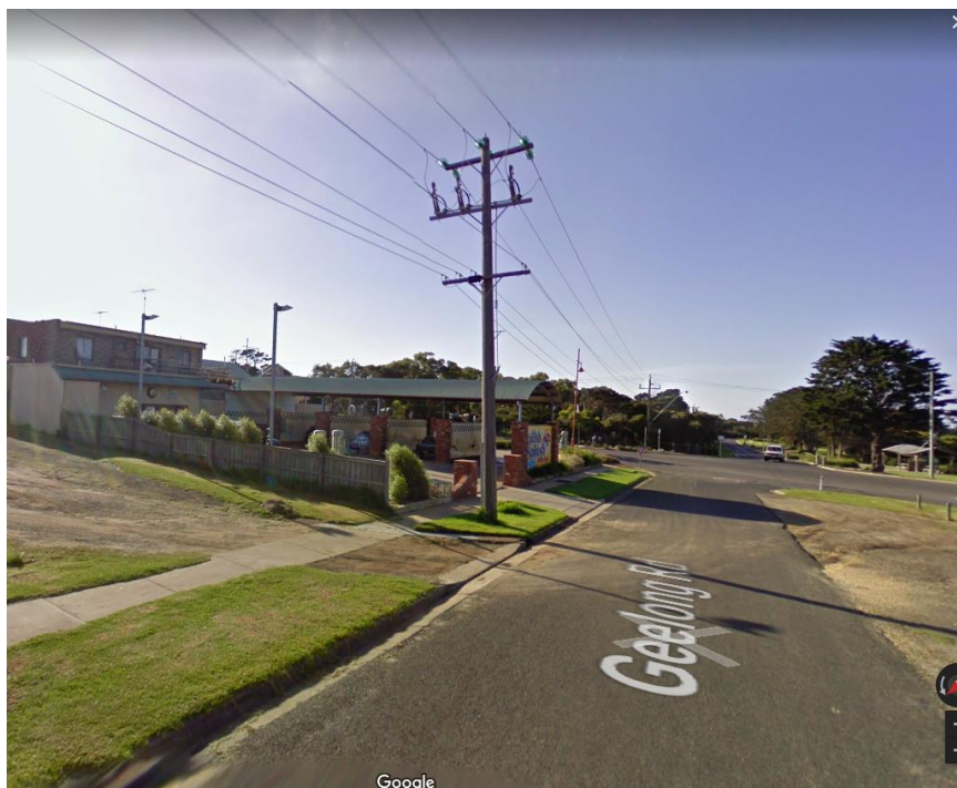
Photo 8 – Geelong Road road reserve
