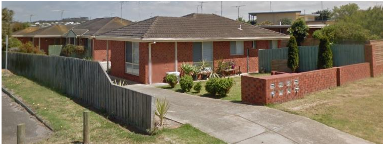
Photo 2 – 5 Rudd Avenue. Source: Google street view
