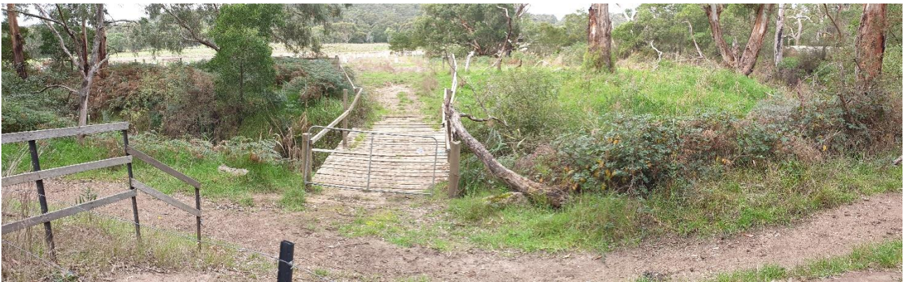
Figure 6 - Picture of existing bridge looking east
