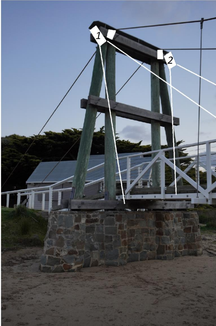
Sketch C) Fixtures 1 & 2 additional installation focused on bridge span proper. Pole downlights shown for position only
