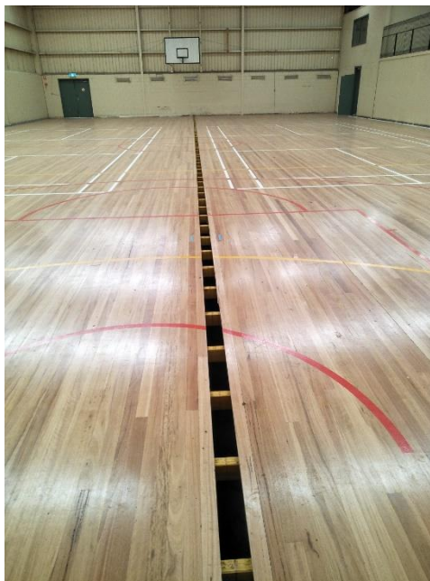
Centre boards removed to allow for expansion and to be replaced with additional expansion joints/boards
