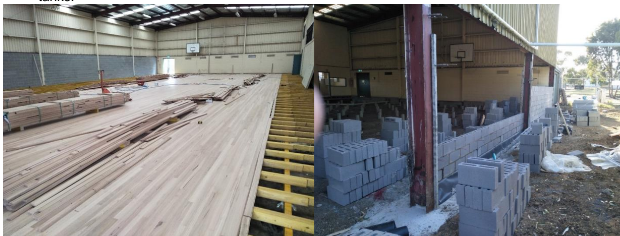
Replacement of sub-floor, flooring and blockwork wall
