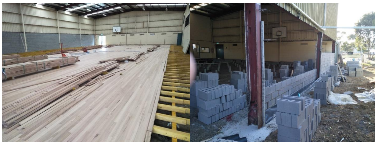
Replacement of sub-floor, flooring and blockwork wall
