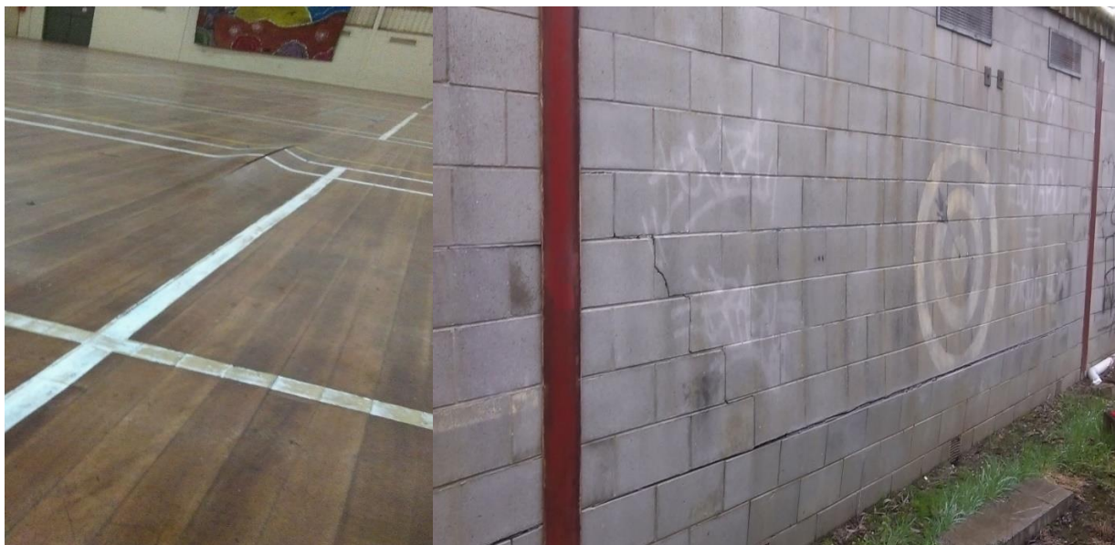
Buckling in flooring and movement in blockwork wall
