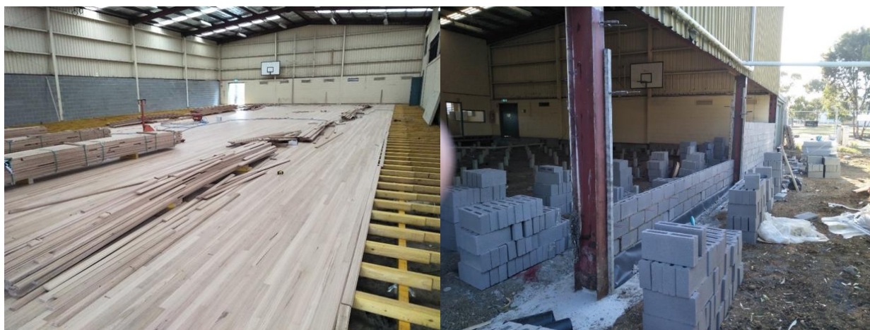
Replacement of sub-floor, flooring and blockwork wall
