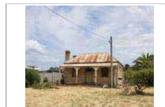
The Cottage , 14 William Street, Port Fairy (VHR H2078) is significant as an intact example of a simple timber dwelling from the late 1840s or early 1850s and its potential, due to its good condition and lack of modifications since completed, to inform our knowledge of construction methods, timbers, hardware, materials and decorative finishes from the mid nineteenth century.
