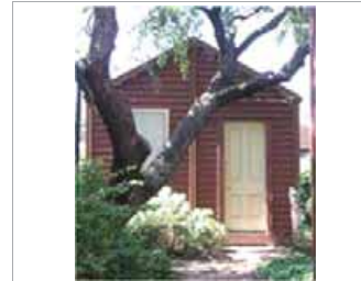
The Bellhouse Iron House , South Melbourne (VHR H1888) is significant as one of the few surviving examples of prefabricated, portable iron housing imported from England in the 1850s due to the rapid increase in population and scarcity of materials and labour during the gold rush.
