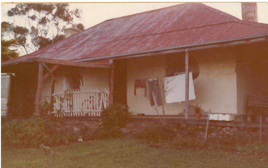
At one stage the facade was rendered. Render has now been removed with some traces still evident. (Image: https://vhd.heritagecouncil.vic.gov.au/places/69772 )
