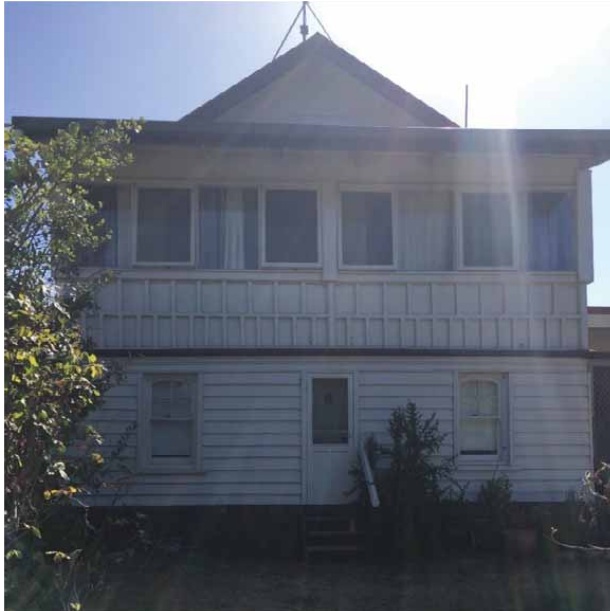
Primary elevation of 'Scammell' (now facing the rear of the site) (Source: Vicki McLean 27.02.19)
