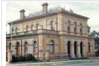
Stawell Court House, Stawell (VHR H1997) built in 1878-79 is significant as a particularly fine and highly intact example of a large court house in the Victorian Free Classical style. It incorporates the key features of a recessed entry, arcade, gallery and hipped roof.
