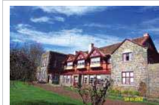
The Murndal Homestead , Tahara (VHR H0289) is significant as a particularly fine and highly intact example of a large-scale pastoral enterprise in Victoria. The place exemplifies the pattern of land settlement during the nineteenth century.
