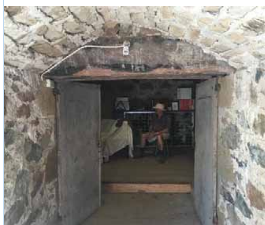
View to deep timber lintel and double doors at cellar threshold. (Image: Vicki McLean 27.02.19)
