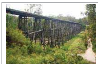
Rail Bridge over Stony Creek, Nowa Nowa (VHR H1436) is significant as a fine example of a timber trestle railway bridge, demonstrating the ingenuity and skill involved in constructing a railway line over a long distance, through difficult terrain and utilising local timber resources.
