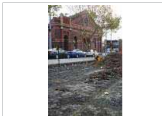
The Cable Tram Track Formation , North Melbourne (VHR H0988) is the only known cable tram track to survive intact in Melbourne and has the potential to contain subsurface evidence of the connection between the engine house and the underground cable tunnels and the track arrangement for the shunting operations.
