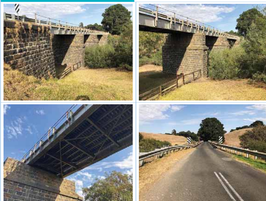
Pollocksford Bridge (from top left, rotating clockwise): 1. West side of bridge looking north east showing bluestone abutment in the foreground. 2. West side of bridge looking north east showing bluestone piers. 3. Underside of bridge showing recent decking. 4 West side of bridge looking north east showing asphalted decking. (Source: Ecology and Heritage Partners Pty Ltd 2019)
