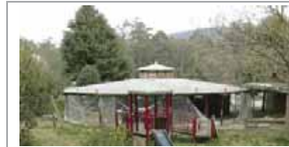
The former Cockatoo Kindergarten (VHR H2303) was used as a refuge for residents of Cockatoo during the devastating Ash Wednesday bushfires of 1983. It has significance for its ability to resonate with other fire-affected communities and the wider Victorian public and interpret to them the experience of 'seeking refuge from fires'
