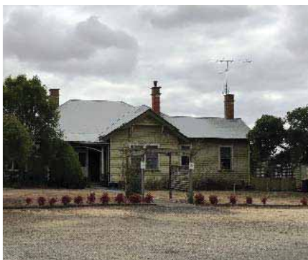
West elevation of the Manse (Source: Ecology and Heritage Partners 2019)
