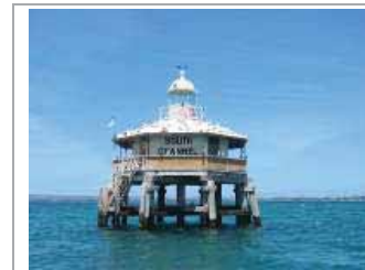
The South Channel and West Channel Pile Lights (VHR H1518 & H1519) are examples of the four manned pile lights that originally serviced ships entering Port Phillip Bay. These were integral to navigational operations along the South and West channels of Port Phillip Bay at a time of heavy traffic in shipping and when passage by sea represented the major form of transport to Melbourne from overseas and interstate.
