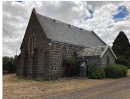
South-east elevation of church (Source: Ecology and Heritage Partners 2019)
