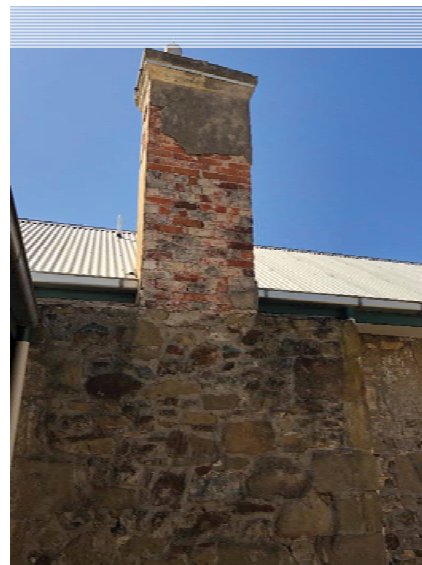
Original chimney showing remnant render over the brickwork at the rear of the original building. (Source: Ecology and Heritage Partners 2019)
