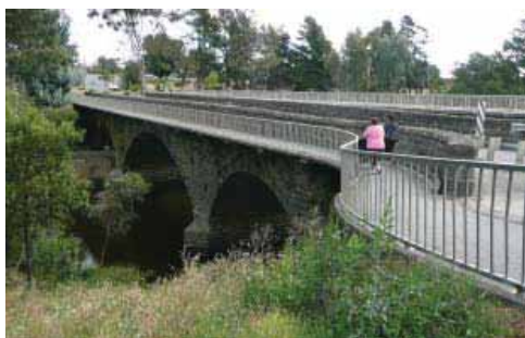
Winchelsea Bridge (Source: hermes.heritage.vic.gov.au )
