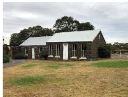
Slaughterhouse – now serving as accommodation (Source: Ecology and Heritage Partners 2019)
