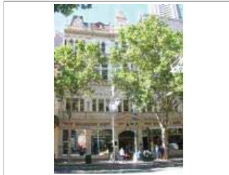
The Salvation Army Temple, Melbourne (VHR H0436) is significant for its enduring association with the Salvation Army, one of the most recognised religious and charitable groups in Australia. The Temple continues to serve as a centre for worship, meetings and the administration of service delivery by 'the Salvos'.
