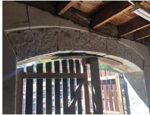
Stone arched opening viewed from inside the stables. (Source: Ecology and Heritage Partners Pty Ltd)
