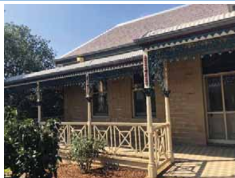
East end of the façade showing original verandah floor, door opening and double hung sash windows. (Source: Ecology and Heritage Partners 2019)
