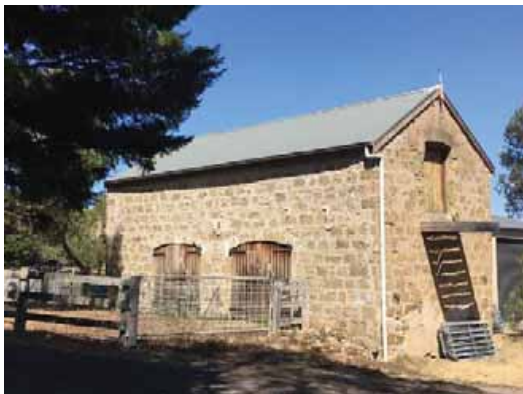
Two pairs of slatted timber doors sit within the arched openings on the east side. North elevation has a timber warehouse style door leading out from the mezzanine. (Source: Ecology and Heritage Partners Pty Ltd)
