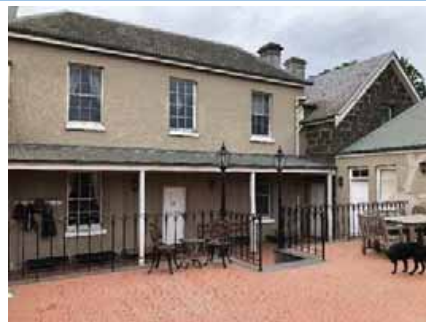
Rear south elevation of the Homestead. (Source: Ecology and Heritage Partners 2019)
