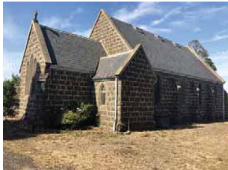
North-west elevation with small gable addition in the foreground. (Source: Ecology and Heritage Partners 2019)
