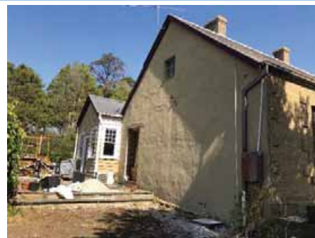
Foymount Homestead, east elevation and addition to the rear. (Source: Ecology and Heritage Partners 2019)
