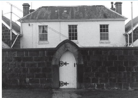
Rear south elevation of the Homestead with bluestone wall that encloses the courtyard in the foreground (Source: State Library of Victoria Pictures Collection)
