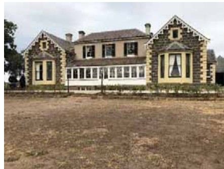
Primary north elevation of Wormbete Homestead. (Source: Ecology and Heritage Partners 2019)
