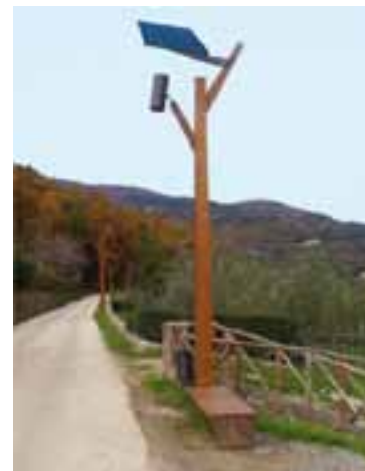
In the long term replace lighting poles
