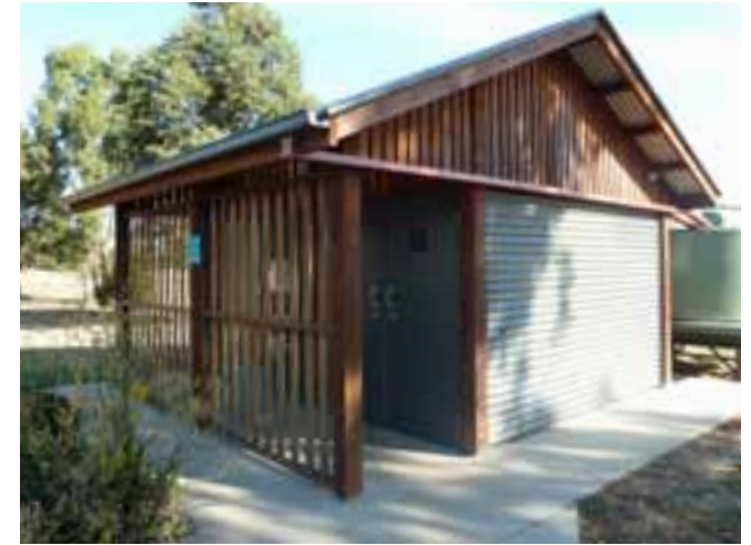
New public toilet facilities in Ararat Rural City Council, Victoria
