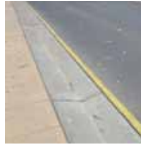
Precast concrete kerbing and asphalt carriageway
