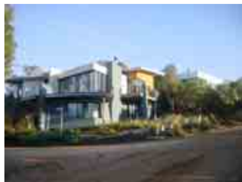
Large building footprint causes building to dominate streetscape and leaves little space for planting of vegetation on the site
