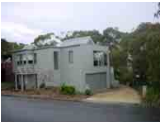
Building has inadequate setback to the street – appears dominant in the landscape
