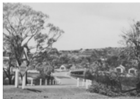
Original Anglesea Bridge
