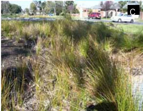
C: Example of Water Sensitive Urban Design (WSUD) which can be incorporated into on street car parking area.
