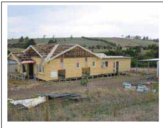
Dwelling under construction in Deans Marsh
