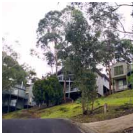
Figure 16: No Front Fencing
