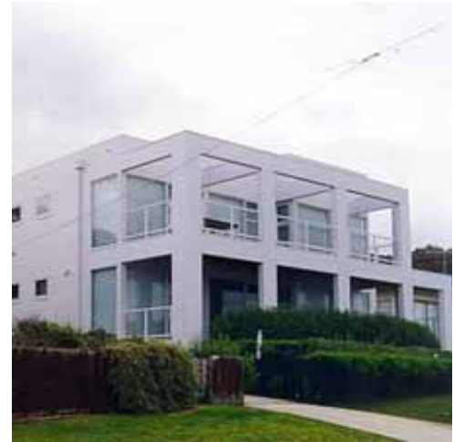
Figure 13: Inappropriate Building Styles Appear throughout Lorne
