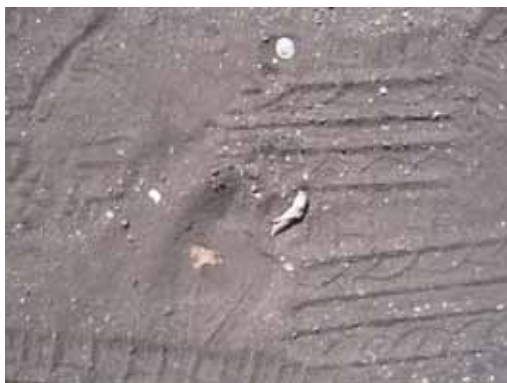
Parking on a midden adjacent to Inlet Crescent. The parking area and paths need to be redefined.
