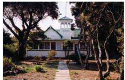
One of the few remaining historic buildings in Torquay, which is rated as highly contributory to neighbourhood character
