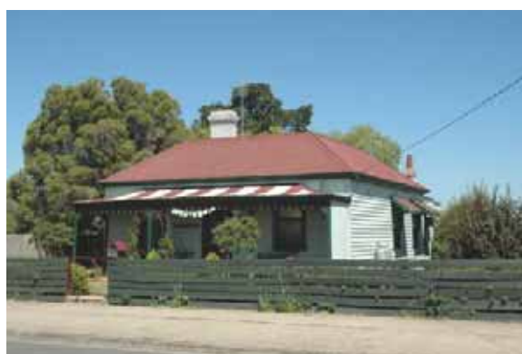
Figure 8.22: Former Police Station, Main Street, Winchelsea, 2008. Source: Wendy Jacobs.
