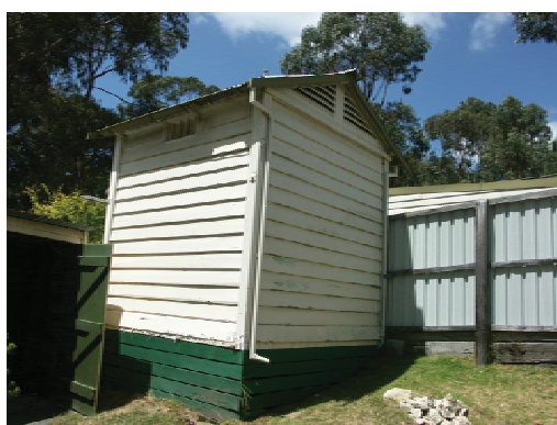
Figure 8.21: Police Lock Up, Smith Street, Lorne, 2005. Source: David Rowe.
