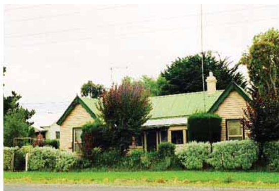
Figure 5.09: Former Deans Marsh Hotel, Deans Marsh, c.1998. Source: Context Pty Ltd.
