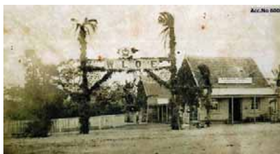
Figure 5.01: Original Barwon Hotel, 1867. Source: Winchelsea & District Historical Society Inc., image 6005s.
