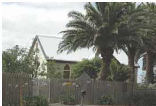
Figure 8.05: Former St. Saviour's Anglican Church, Modewarre, 2008. Source: Wendy Jacobs.
