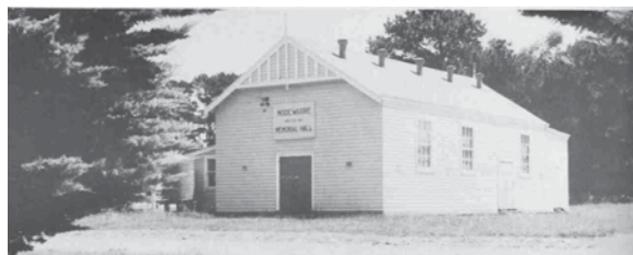
Figure 8.31: Modewarre Memorial Hall, c.1965. Source: Shire of Barrabool Centenary 1865-1965.
