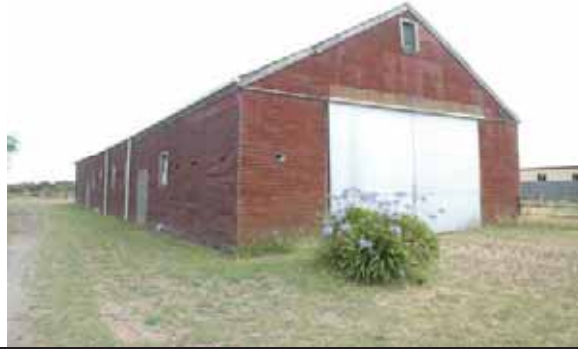
Figure 6.08: Former P1 Army Hut from the Gherang Army Camp, now located in Barkly Street, Winchelsea, 2008. Source: Wendy Jacobs.
