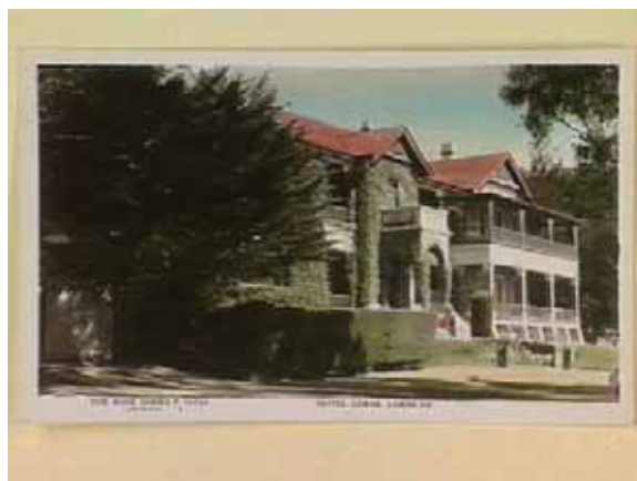
Figure 7.22 Lorne Hotel, c.1925. Source: La Trobe Picture Collection, State Library of Victoria, accession no. H90.160/110, image no. a01686.
