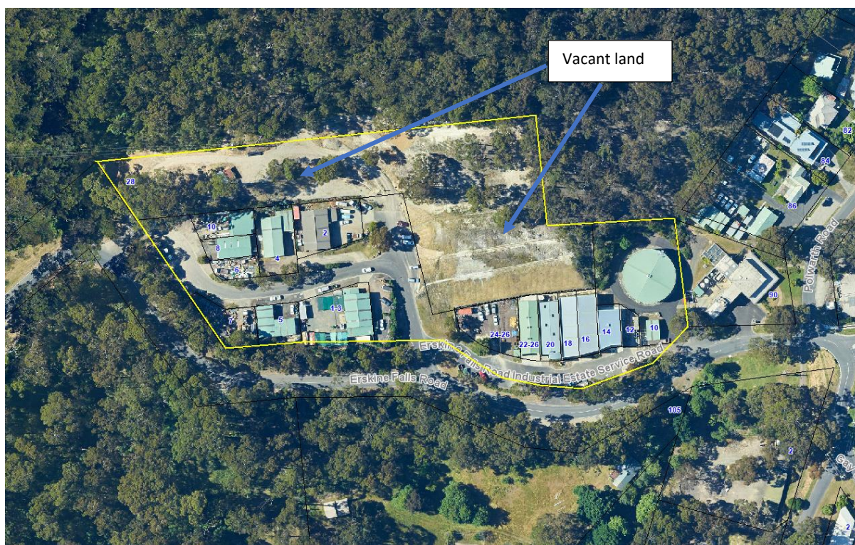
Figure 13: Lorne Industrial Precinct
