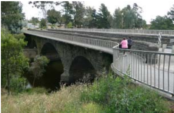
Winchelsea Bridge (Source: hermes.heritage.vic.gov.au)
