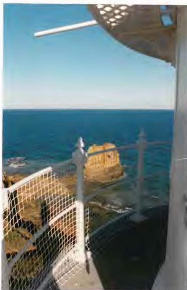
*Figure 28 The exterior gallery, with original cast iron balustrading and recent mesh infill.*
