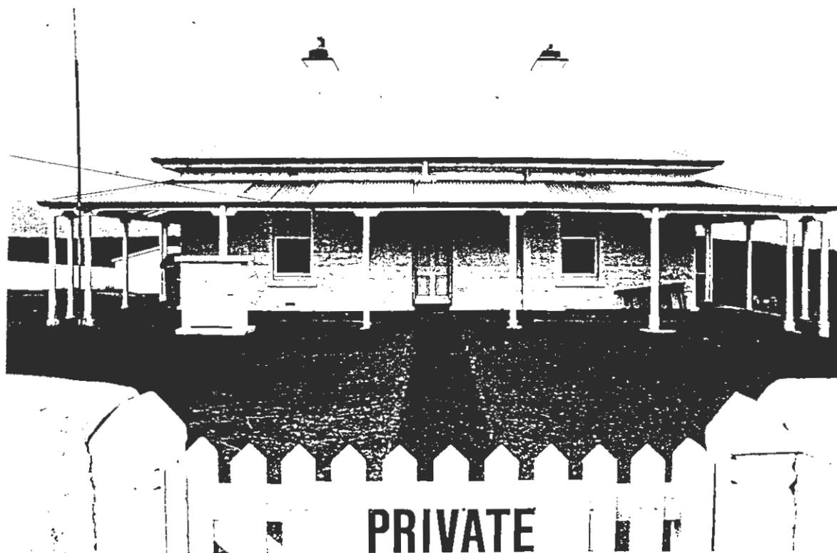
Figure 39 Cape Nelson Lighthouse Keepers' Cottage. Note the timber verandah posts and carved timber brackets. Reproduced from Cape Nelson Lightstation.
