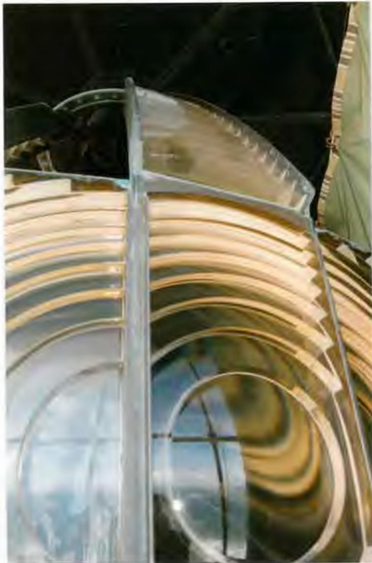
*Figure 46 Cape Otway lantern interior, with original Chance Bros. optic lens.*
