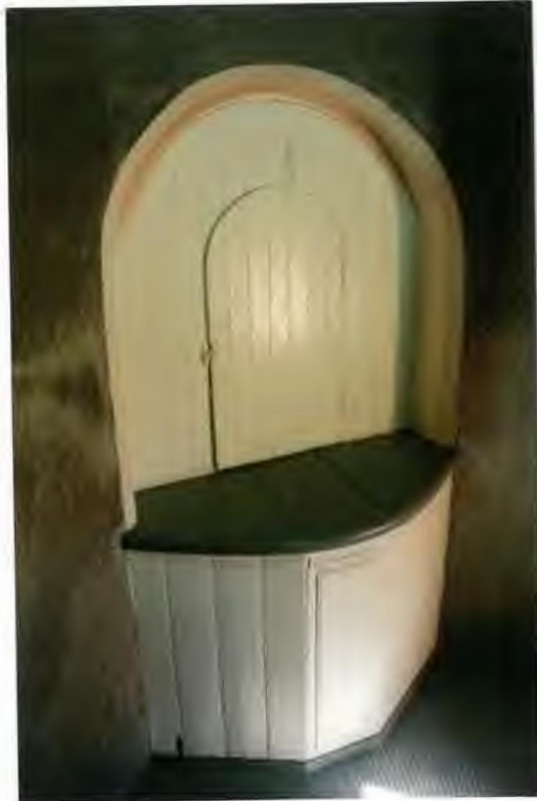
*Figure 26*      *The door opening to the auxiliary light at first landing level. The auxiliary light was discontinued in 1919.*
