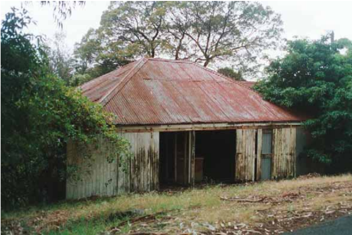
Photo 1.26: Upper Kincaig outbuilding, 127-129 Smith Street. SIGNIFICANT heritage place.
