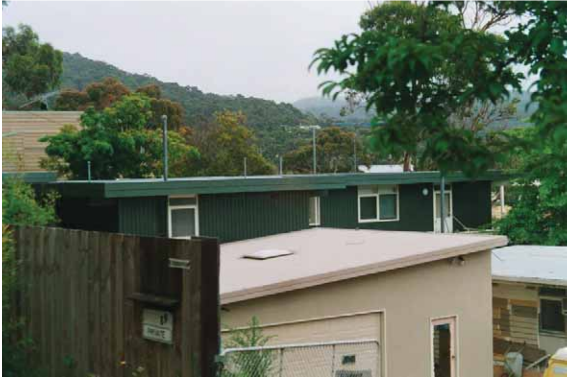
Photo 1.19: House, 87 Smith Street. COMPATIBLE place.
