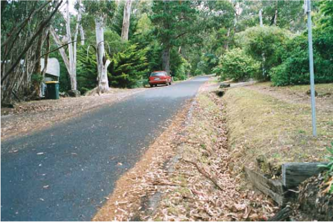
Photo 1.45: Beal Street (from Mountjoy Parade) showing grassed verges and open spoon drains. Also note the lack of formal footpaths.
