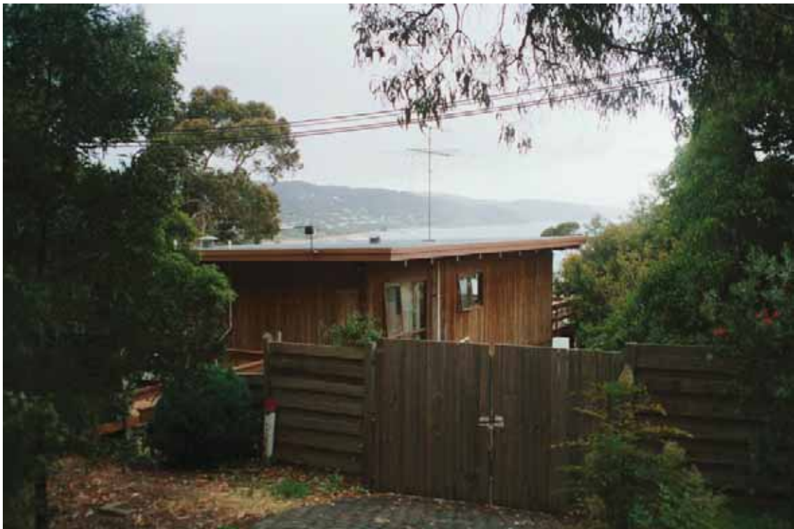
Photo 1.18: House, 71-73 Smith Street. COMPATIBLE place.
