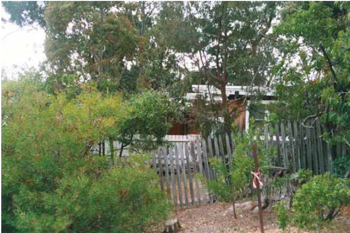
Photo 1.24: House, 119 Smith Street. COMPATIBLE place.
