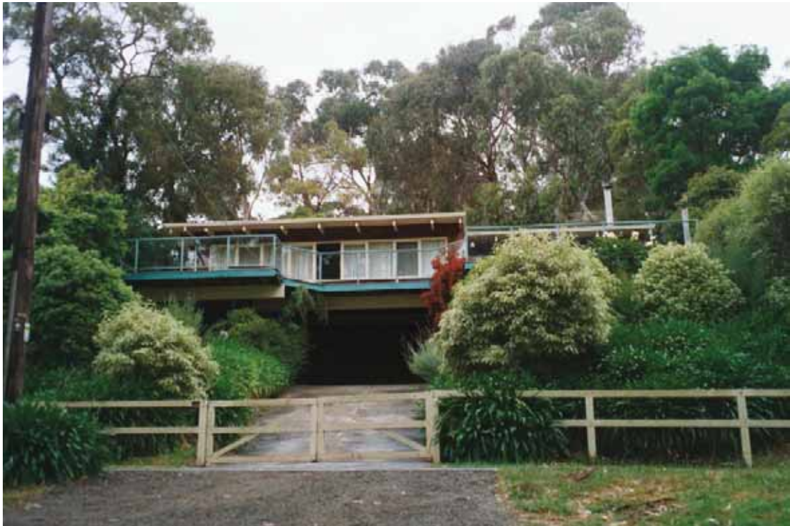
Photo 1.13: House, 234 Mountjoy Parade. SIGNIFICANT heritage place.
