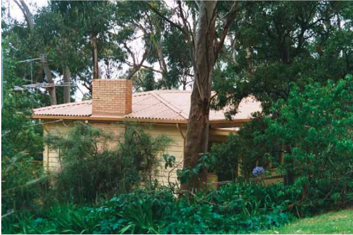
Photo 1.27: House, 137 Smith Street. COMPATIBLE place.
