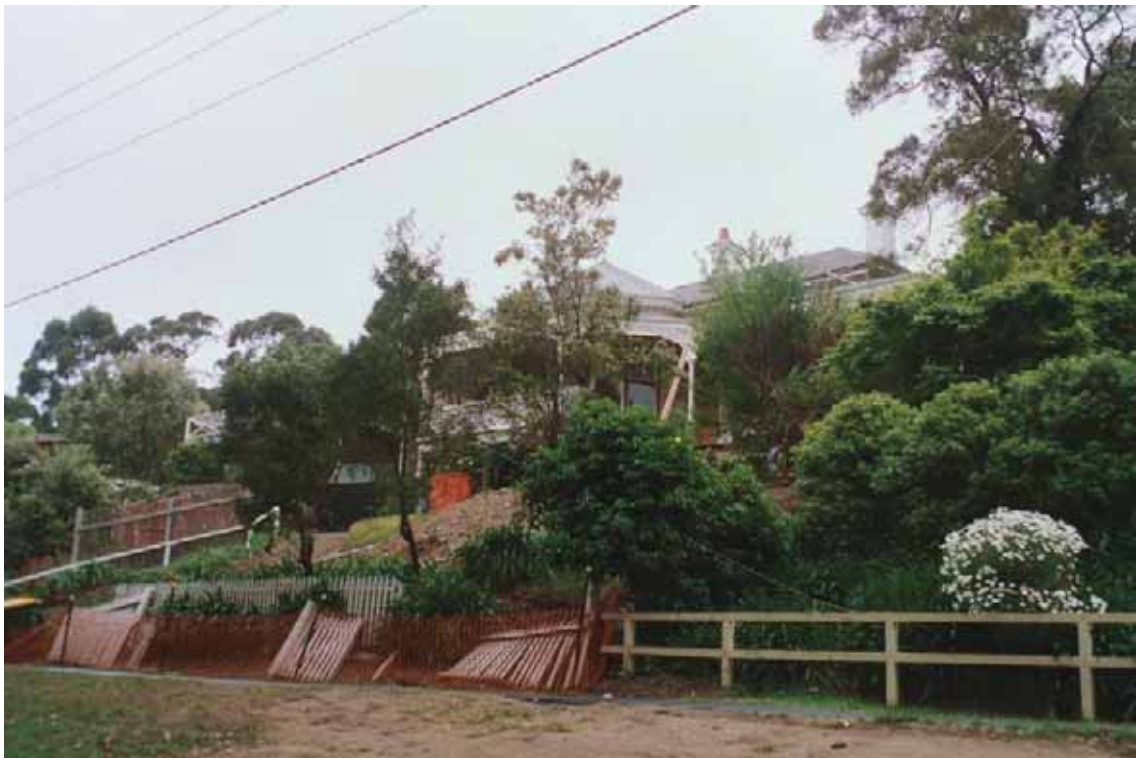
Photo 1.14: Lower Kincaig, 236 Mountjoy Parade. SIGNIFICANT heritage place.
