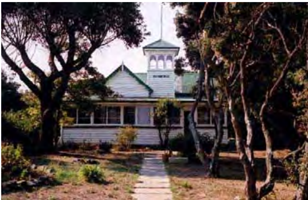
Figure 3: Historic House in Neighbourhood Three with Mature Vegetation
