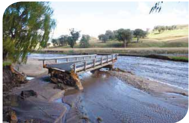
Bridge on Guys Forest Road, Burrowye (after flood, 2012). Courtesy Towong Shire Council
