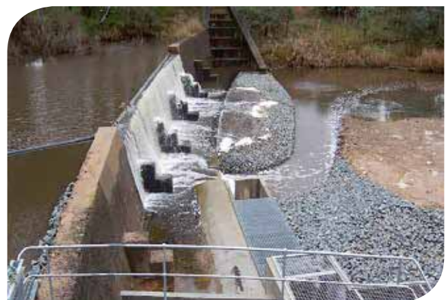
Structure allowing fish movement past a weir. Courtesy DEPI
