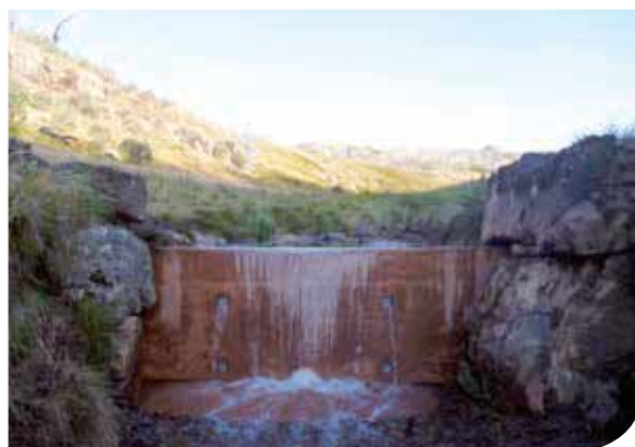
Artificial barrier installed to protect the Shaw Galaxias from introduced trout. Photographer: Michael Nicol
