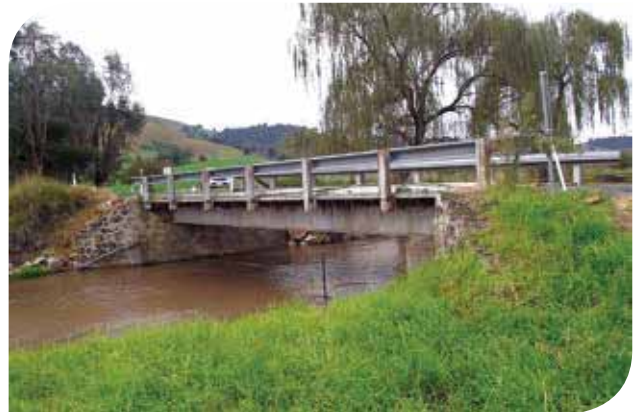
Bridge on Guys Forest Road, Burrowye (before flood). Courtesy Towong Shire Council
