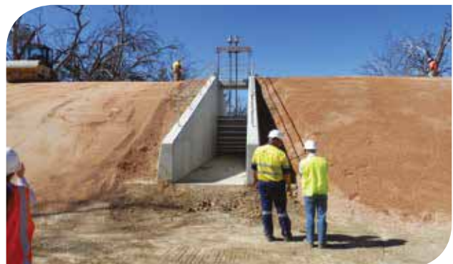
Hattah Lakes Wetlands. Environmental watering regulator gate. Courtesy Mallee CMA
