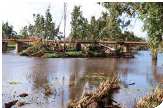
Piled up debris against a bridge on the Loddon River following the 2011 flood. Courtesy DEPI
