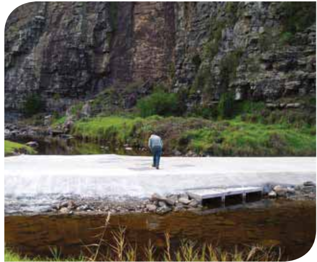
A previous barrier, this road has been adapted to allow fish passage. Courtesy Corangamite CMA
