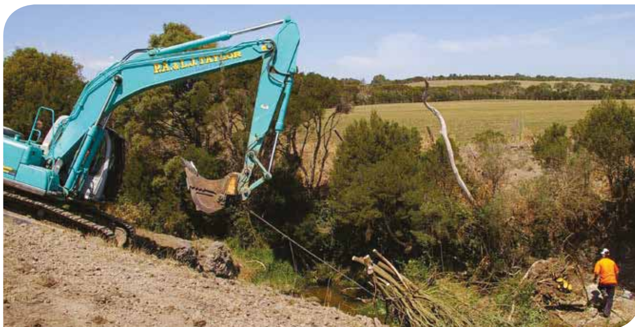
Willow removal works on Fish Creek. Courtesy West Gippsland CMA
