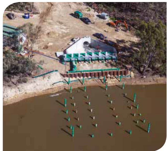
The Messengers pumping station aims to water Hattah Lakes efficiently and maximise ecological outcomes. The Living Murray is a joint initiative funded by the New South Wales, Victorian, South Australian, Australian Capital Territory and Commonwealth governments, coordinated by the Murray–Darling Basin Authority. Courtesy Mallee CMA
