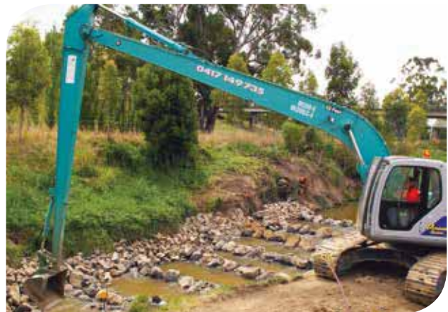
Constructing Tarwin River Fishway. Courtesy West Gippsland CMA
