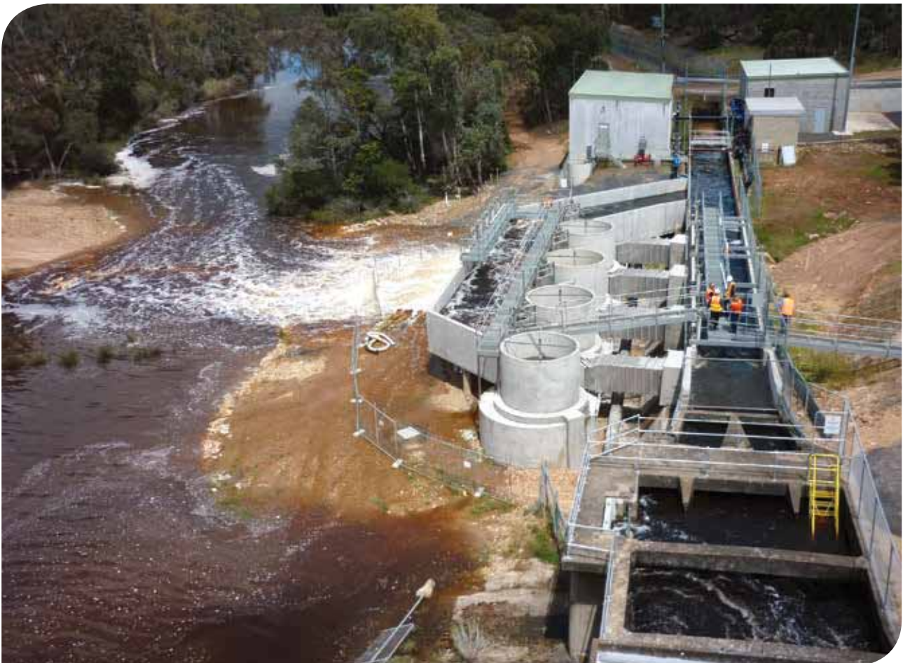
Carp screens and structure to release environmental water to the Glenelg River. Courtesy Glenelg Hopkins CMA
