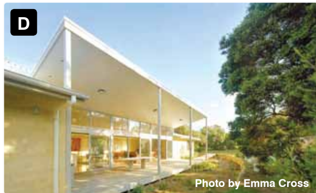
C. Window and door openings for cross ventilation D. North-facing living and outdoor areas with sun protection
