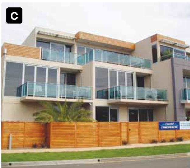
A. Inclusion of lightweight elements to break up bulk B. Example of contemporary townhouse development C. Upper levels stepped in to reduce building bulk D. Varied façade treatment
