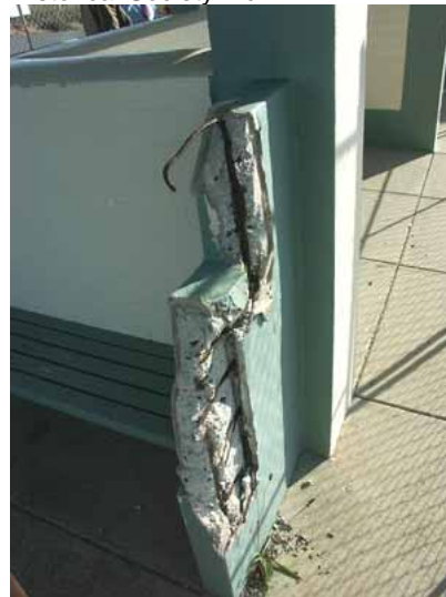
Photo 3.25: Detail of substantially spalled eastern end of south-facing seat.
