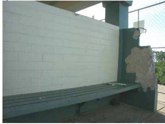
Photo 3.17: Detail of bench seat, south face. Note the substantially spalled concrete end to the seat.
