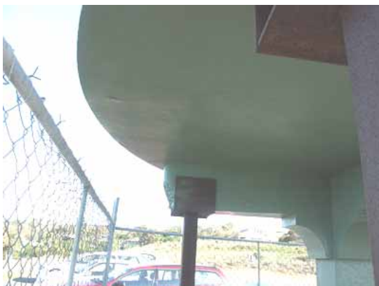
Photo 3.26: Detail of projecting southern portion of the roof showing supporting introduced steel props.
