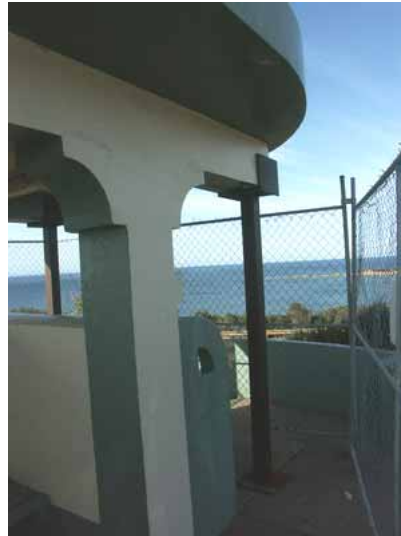
Photo 3.09: Detail of concrete pier and cantilevering beam, south-west corner. Note the temporary steel prop supporting the beam.
