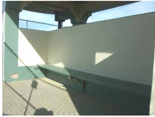
Photo 3.15: Detail of bench seat, east face. Note the missing timber slat to the seat and also the spalled concrete at the base of the column.
