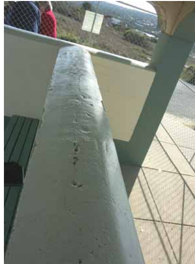
Photo 3.19: Detail of rounded capping to central solid brick wall separating the east and west seats.
