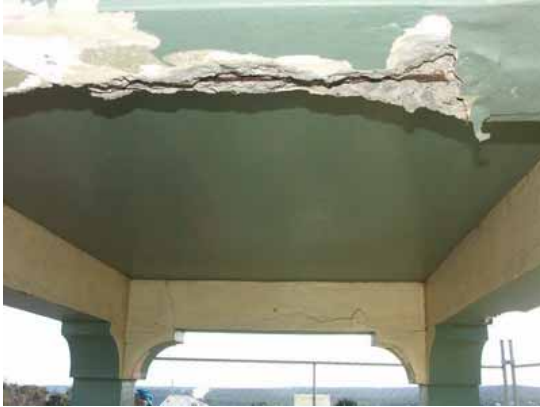
Photo 3.28: Detail of substantially spalled south-facing beam.
