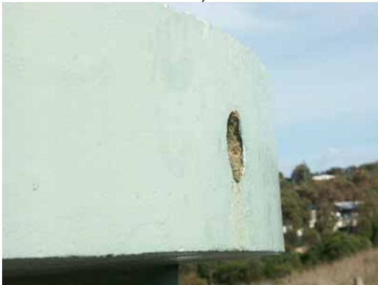
Photo 3.14: Rainwater outlet detail (west roof face).
