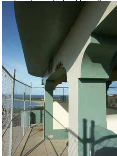
Photo 3.11: Detail of east side, showing columns with curved brackets and widely-projecting roof.
