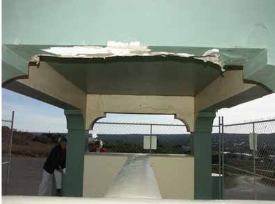
Photo 3.12: View looking west (from the east end) showing spalled beam (foreground) and dividing wall (that acts as a backrest for the bench seating on the east and west faces).
