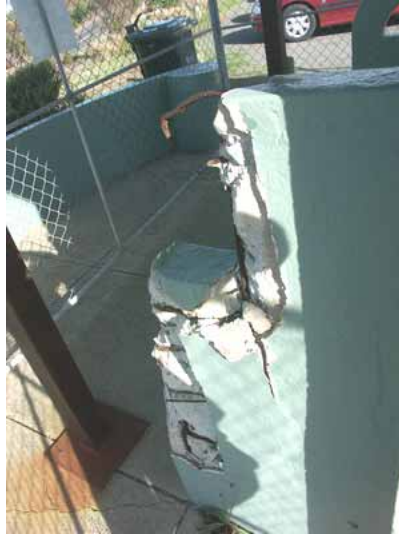
Photo 3.29: Detail of substantially spalled and cracked eastern end to the south-facing seat.
