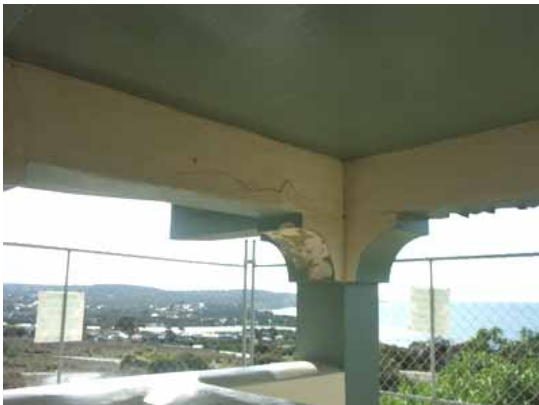
Photo 3.10: Detail of roof soffit and junction of beams with column. Note the cracking in the west beam and spalled bracket to the column.
