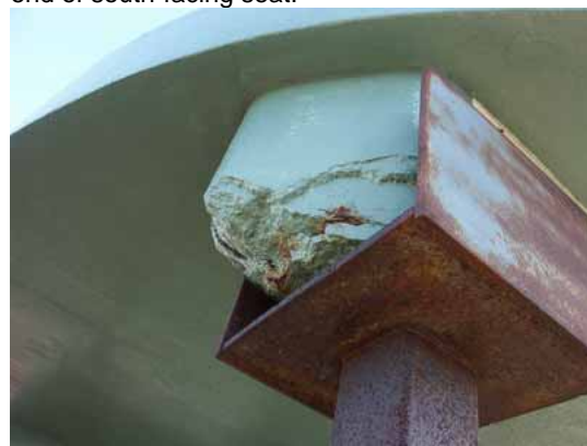
Photo 3.27: Detail of spalled southern end of the east-facing beam supported by an introduced steel prop.
