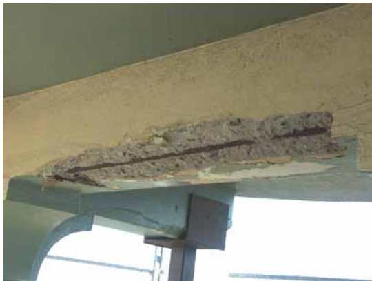
Photo 3.24: Detail of spalled south-facing beam exposing reinforcement.
