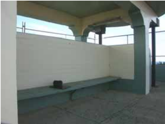
Photo 3.16: Detail of bench seat, west face. Note the solid brick wall that acts as a backrest.
