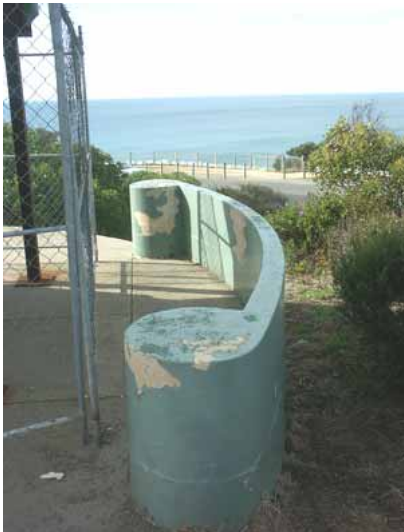
Photo 3.20: Detail of curved balustrade (south end) showing peeled paintwork and spalled concrete.
