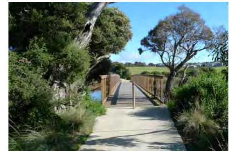
Sealed concrete path and bridge crossing on the Surf Coast Highway
