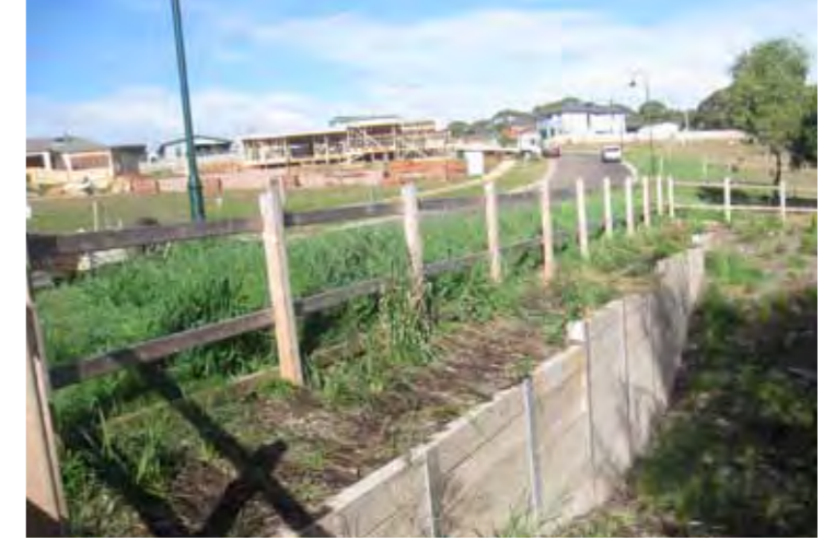
Retaining wall and fence on Spring Valley Drive
