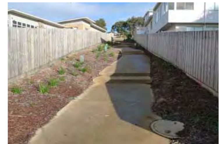
Stepped concrete path access from Ocean Views Estate
