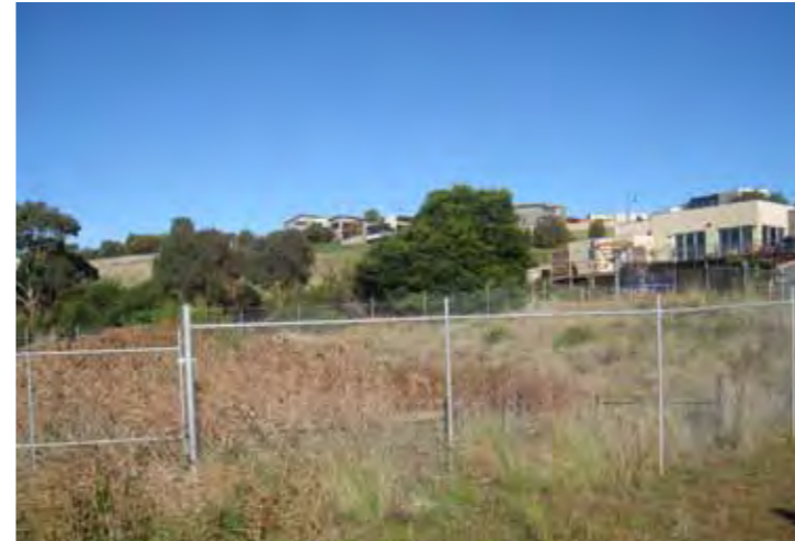
Chainmesh surrounding water treatment facility
