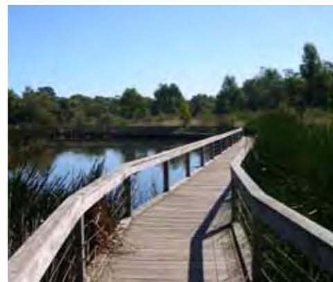
Boardwalk with handrails through wetland.
