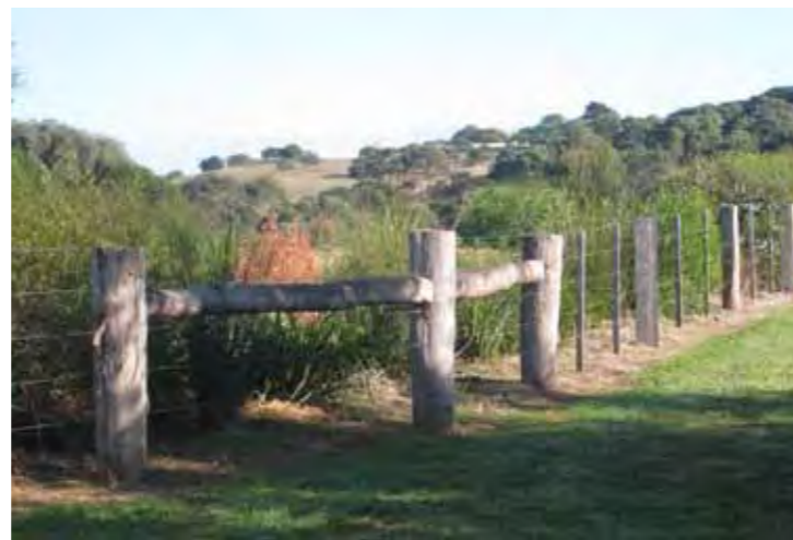
Bike park site fencing
