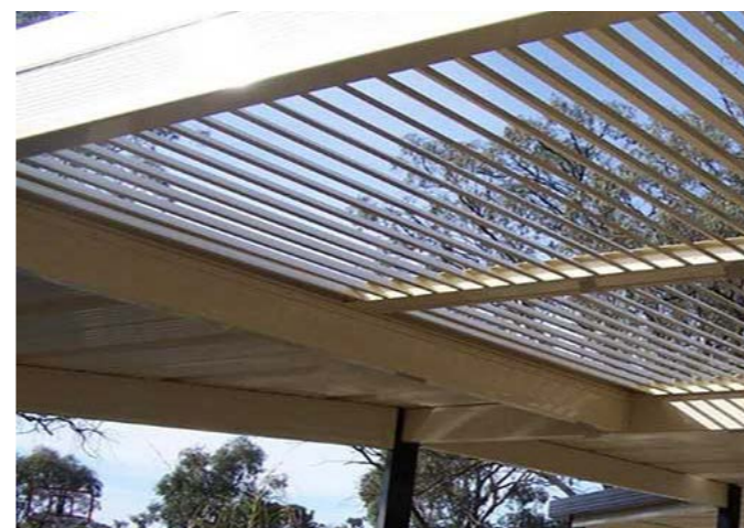
Shade structure over existing deck A shelter/pergola is proposed to be installed over the existing deck to provide shade. Concerns regarding impacts of indoor light levels are to be addressed by having a combination of solid and open roofing materials, with the more open portion being at the western end of the deck near the hall windows. New solid roofing is also proposed on the north side of the building allowing all-weather outdoor play.
