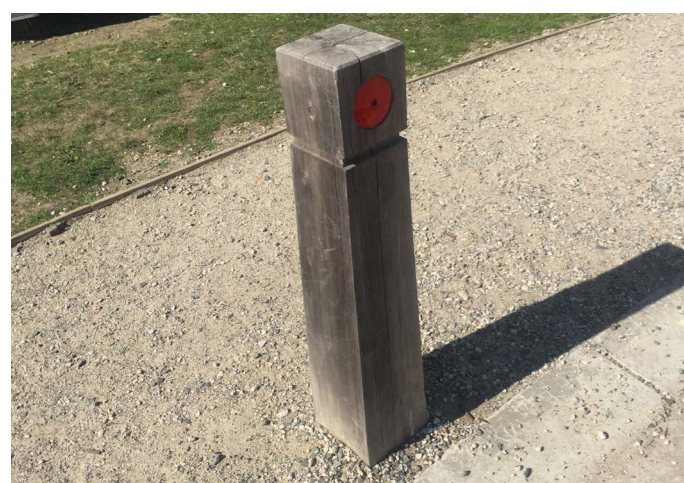
Timber bollards Existing bollards to be retained, separating the car park and pedestrian spaces.
