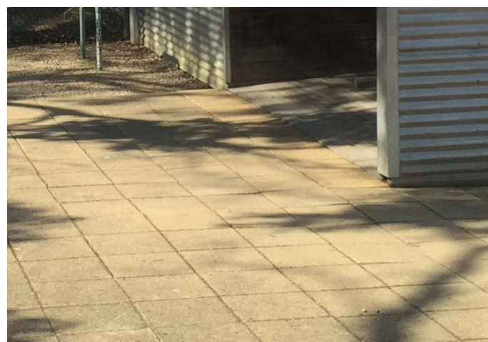
Square concrete pavers Concrete pavers at the existing entry to be retained, and pavers to match used at the proposed new entry.
