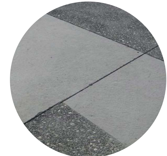
PAVING OPTIONS SANDBLASTED / SAWCUT CONCRETE
