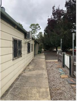
Figure 24- Condensing unit located on façade bracket at high level, installed in 2021
