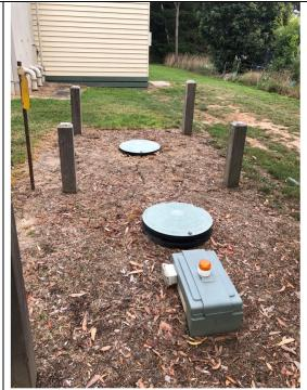
Figure 12- Wastewater treatment system with in ground storage/treatment tanks
