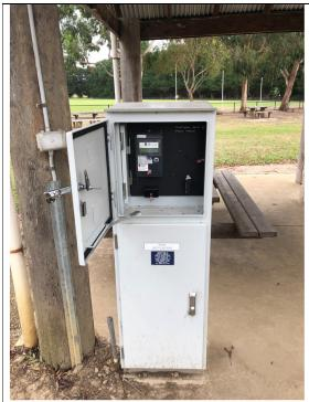
Figure 2- Authority meter panel installed in 2021 located in picnic shelter in Reserve
