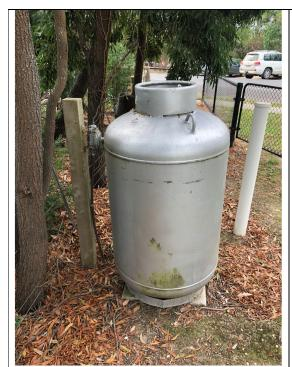
Figure 15- Onsite LP gas storage tank
