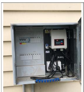
Figure 21- Wastewater Treatment system control panel
