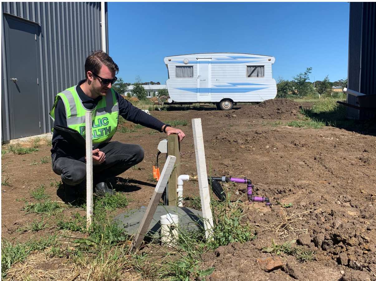
Council's EHO inspecting recently installed pump pit as part of a sand filter system.
