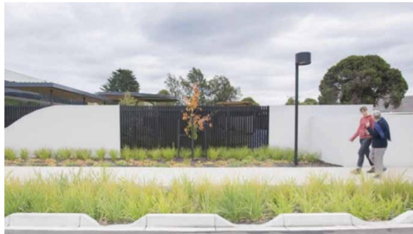
Kerb cut aways at proposed tree locations to enable passive irrigation
