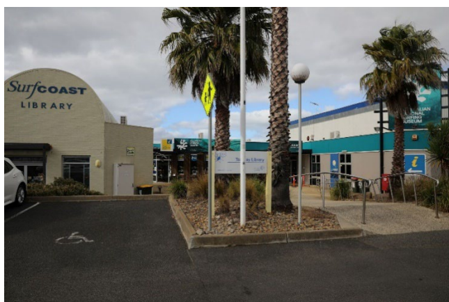
Torquay Library Exterior
