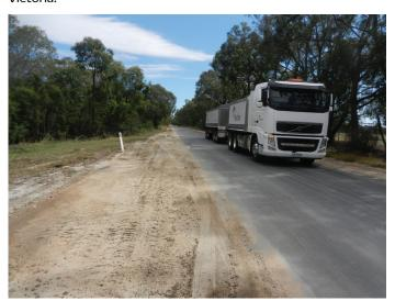
**FOREST AND GRAYS ROADS:** Council has recently completed shoulder widening, pavement strengthening and guardrail installation on a total of about 4km of Grays Road and Forest Road.
