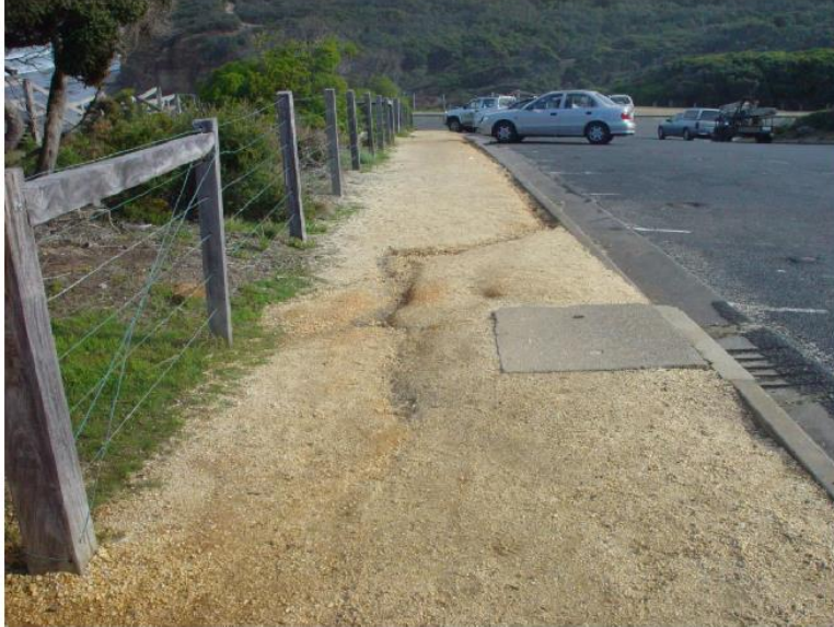
Uneven surface with eroded material flowing downhill to stormwater pits in Hammerhead car park
