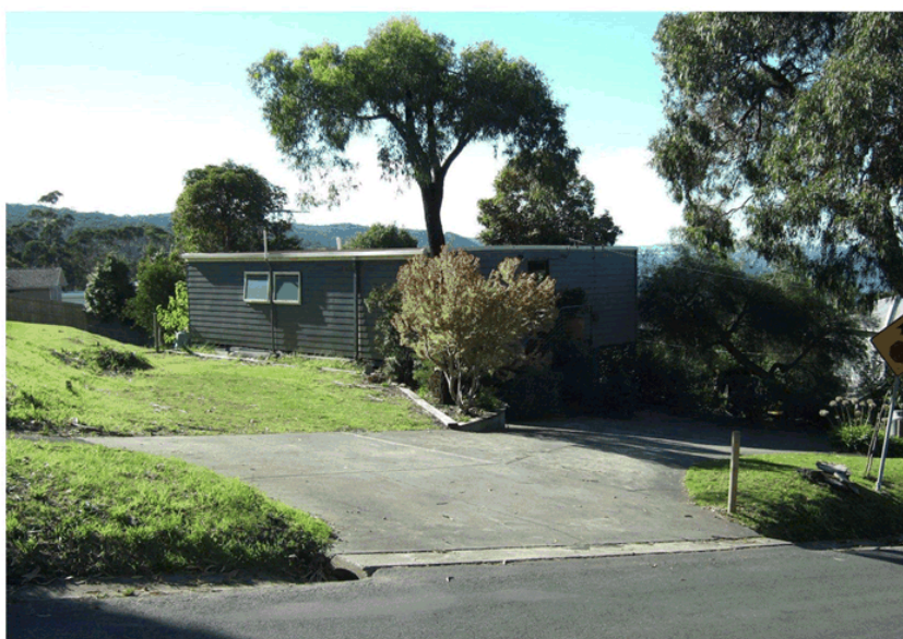
Image 2: Existing 30A crossover and unformed driveway sidling No. 30.
