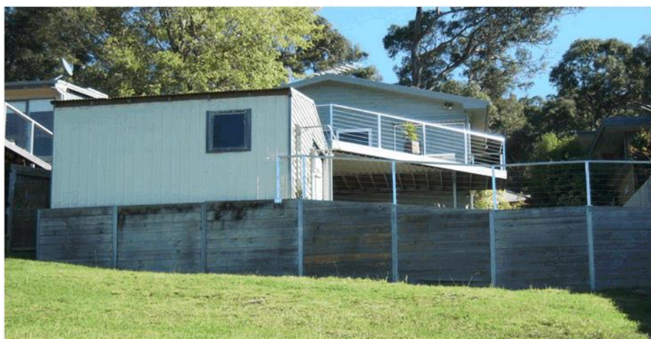
Image 6: 85 Polwarth Rd has a steel shed and timber retaining wall along the west boundary of No. 32.
