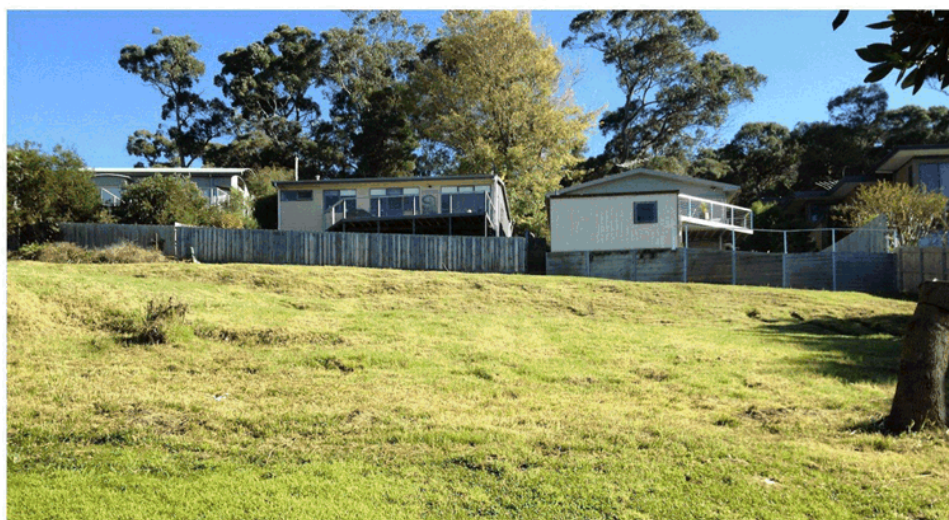
Image 4: The unit 3/34 William St and houses Nos. 87 and 85 Polwarth Rd will continue to share the west boundary of No. 32 William St.
