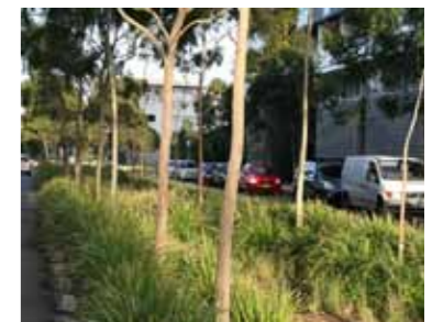
Swale treatment system - car park
