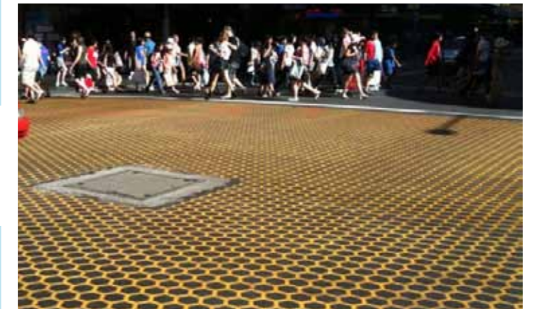
Thermoplastic marking the pedestrian route
