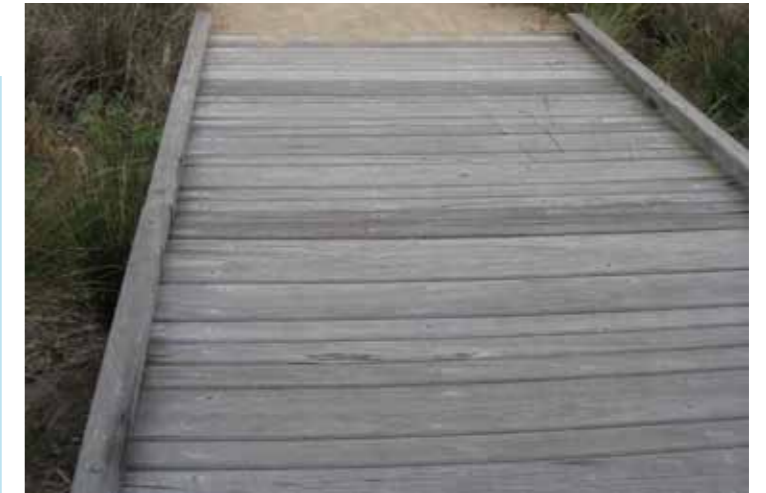
Low key creek crossing / bridge in sympathetic materials
