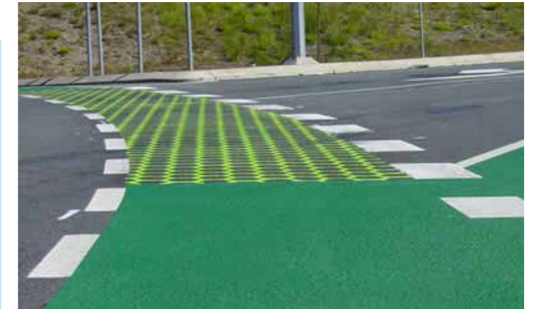
Thermoplastic marking the pedestrian route
