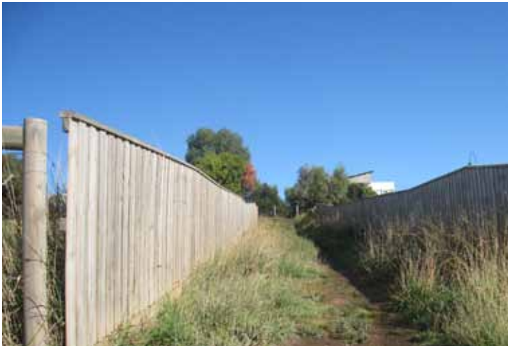
Fencing to private properties and access points
