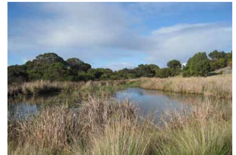
Water treatment facility/wetland to the west of Bowman Track
