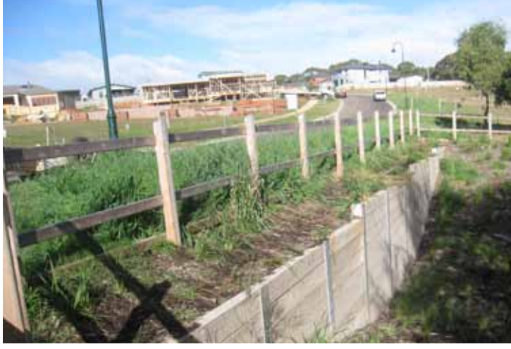
Retaining wall and fence on Spring Valley Drive
