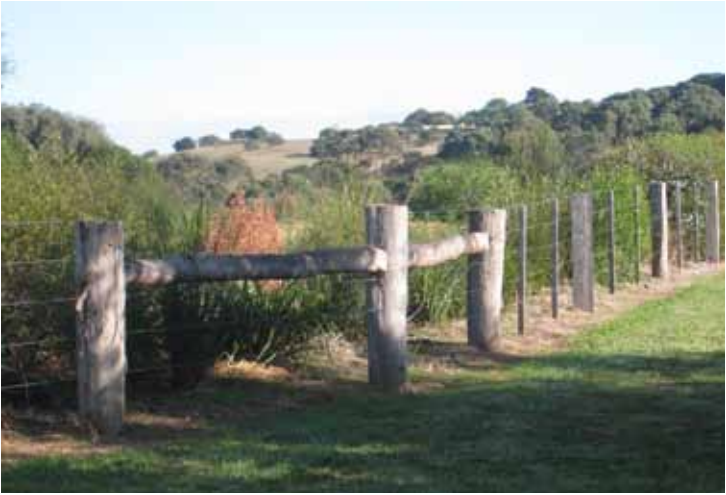
Bike park site fencing
