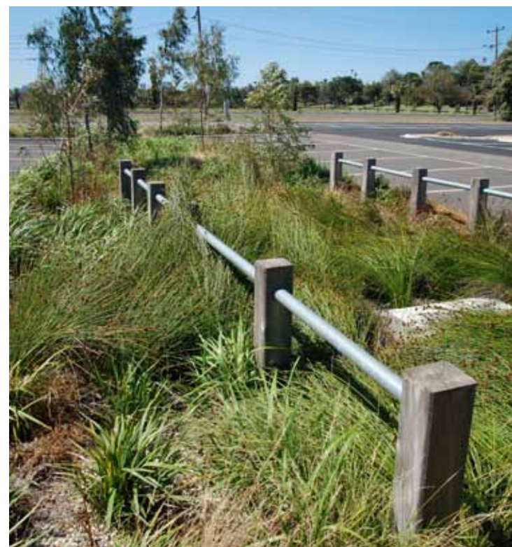
Planted swales to car parks and road edges to treat water prior to run off into creeks and tributaries
