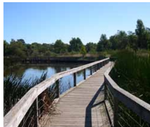
Boardwalk with handrails through wetland.
