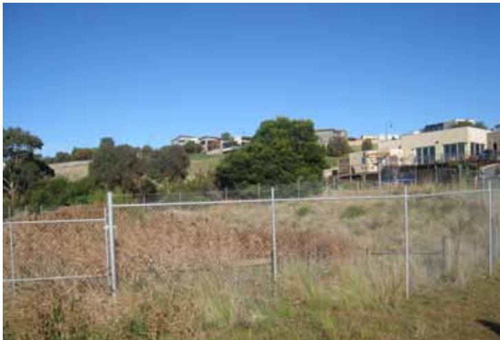
Chainmesh surrounding water treatment facility
