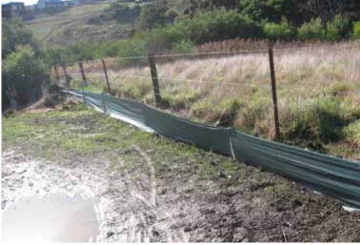
Post and wire fence and silt control at the bike park
