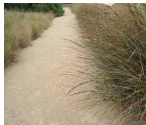
Granitic sand experiential path, in a colour to match the sealed asphalt path
