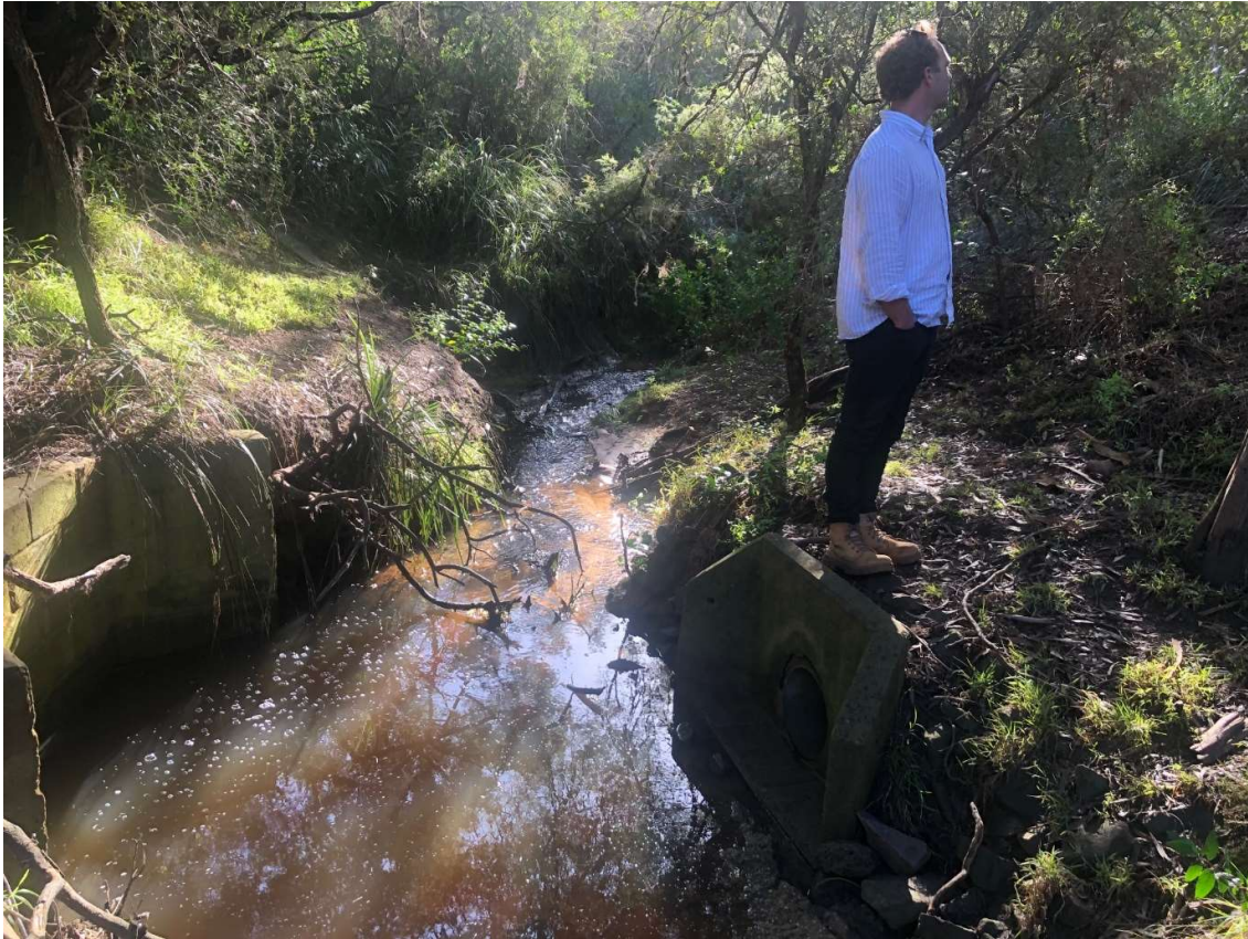
Figure 6 – Existing endwall and pipe outfalls
