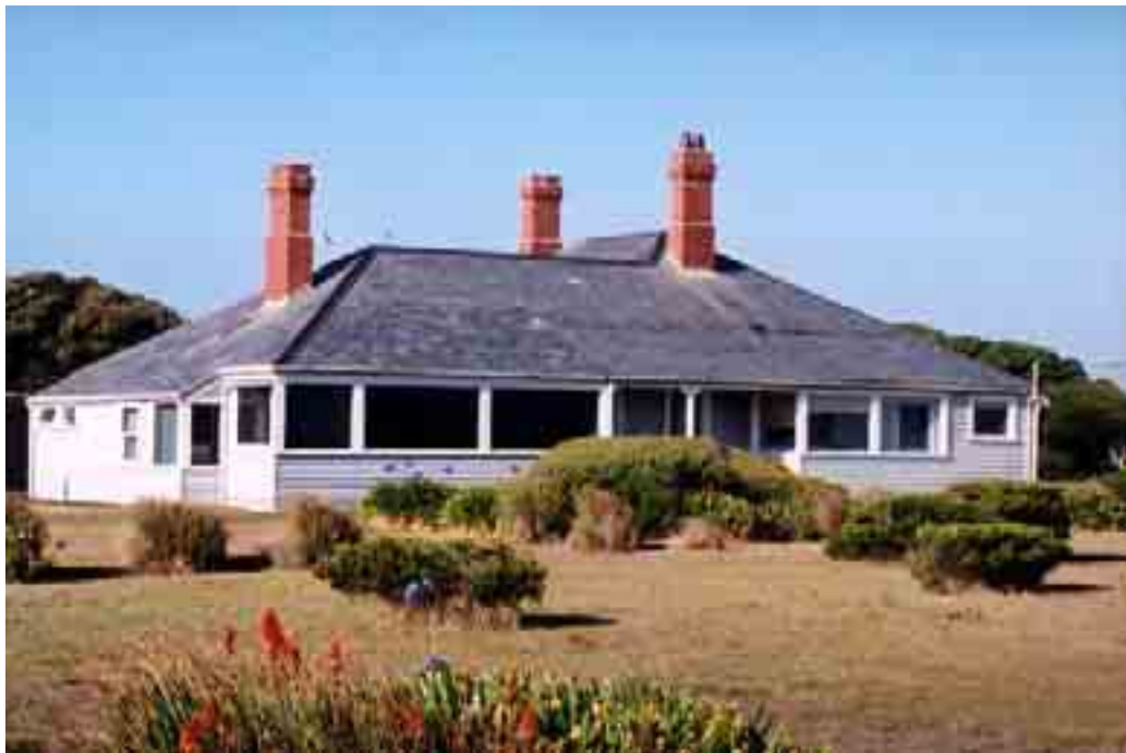
Figure 5: The Lighthouse Keeper's House.
