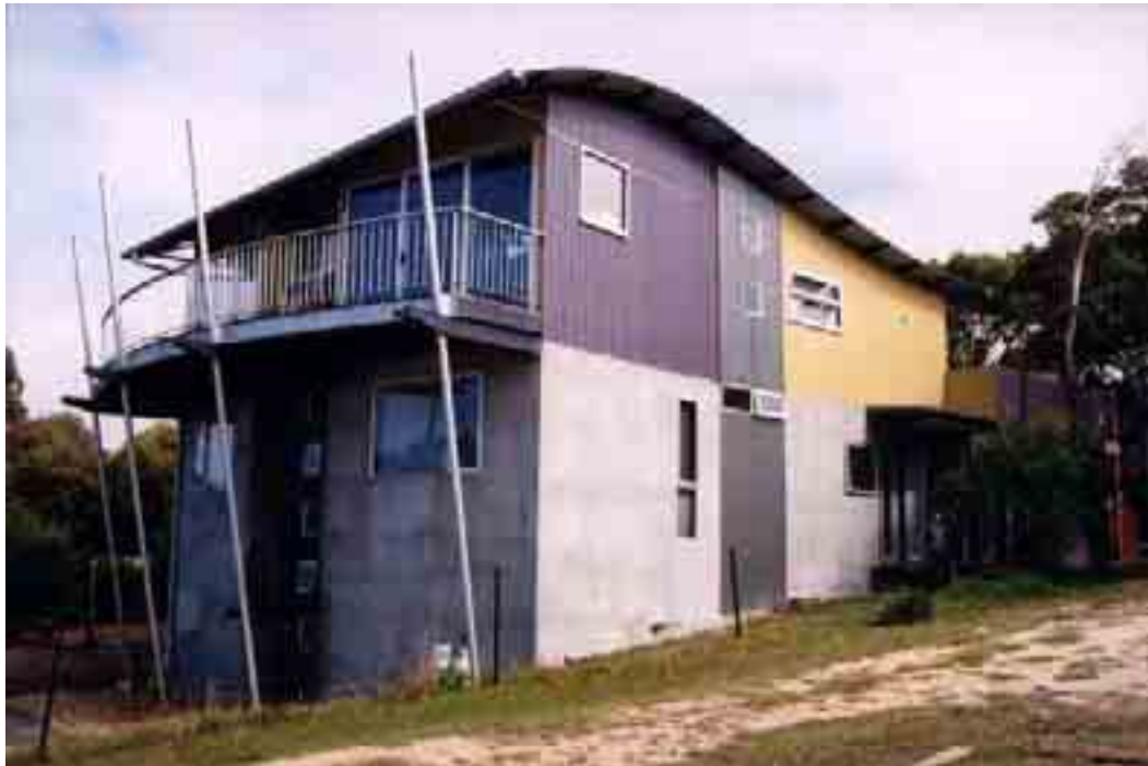
Figure 11: House Rated Most Incompatible with Neighbourhood Character
