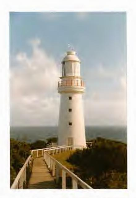
Figure 45 Cape Otway Lighthouse, constructed 1848, with 1891 Chance Bros. lantern.
