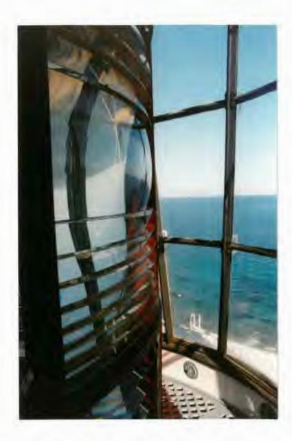
Figure 29 The optic lens at upper lantern level. Note the ventilation covers below the glazing.
