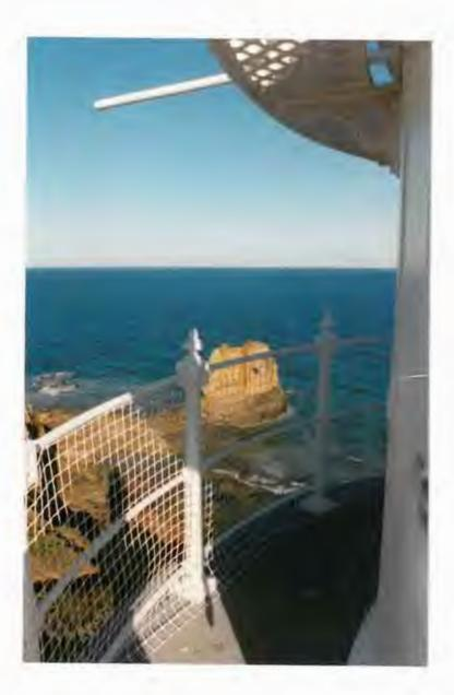
Figure 28 The exterior gallery, with original cast iron balustrading and recent mesh infill.
