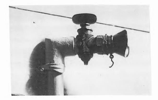
Figure 16 The speaking tube in the head lighthouse keepers cottage (1985). Source: The White Queen.
