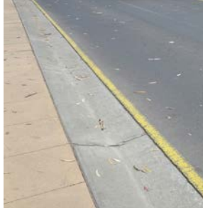
Precast concrete kerbing and asphalt carriageway
