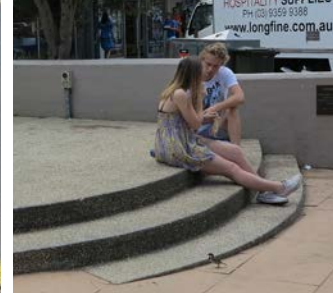
Concrete with exposed aggregate steps and raised platform areas which are used for cafe seating
