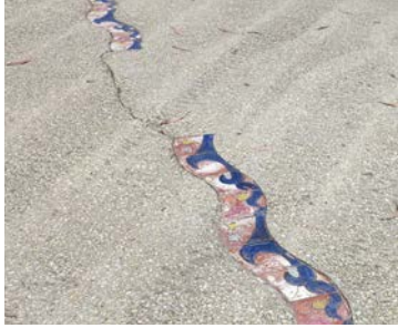
Concrete slab with exposed aggregate is used within the majority of the streetscape. Inlaid decorative tiles are in poor condition.
