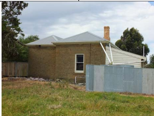
Photo 43: Former manse, west elevation, November 2014.
