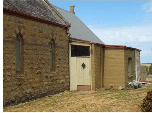
Photo 18: Barrabool Uniting Church, supper room addition, north and west elevations, November 2014.
