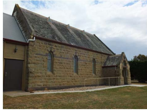
Photo 10: Barrabool Uniting Church, east elevation, November 2014.
