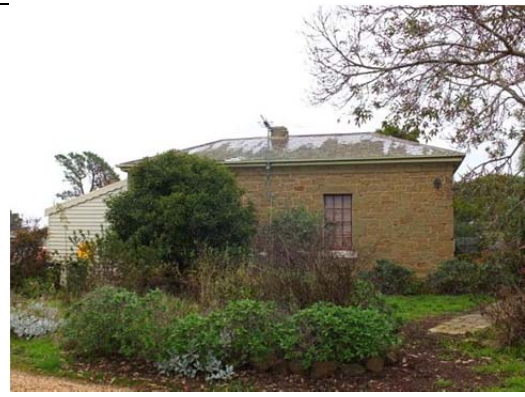
Photo 40: Former manse, east elevation, April 2014.
