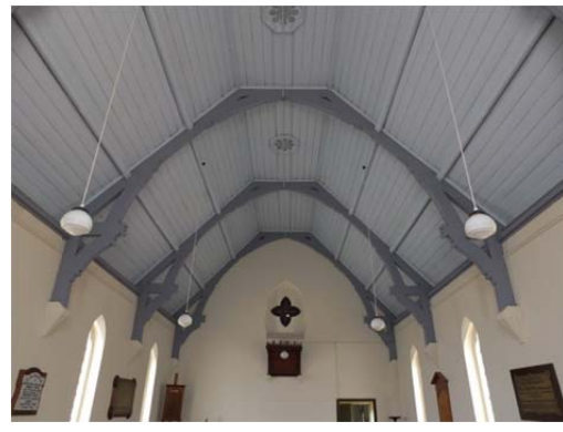
Photo 20: Church interior looking south, view of ceiling, November 2014.
