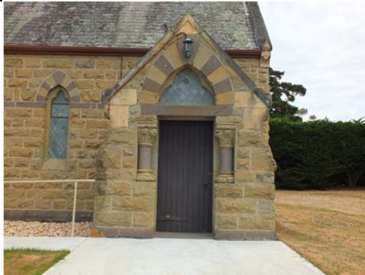
Photo 11: Barrabool Uniting Church, porch detail (east elevation), November 2014.
