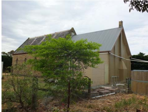
Photo 17: Barrabool Uniting Church & Sunday School Room addition, west and south elevations, November 2014.
