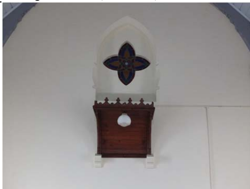
Photo 31: Church interior, detail of pulpit canopy, south end, November 2014.
