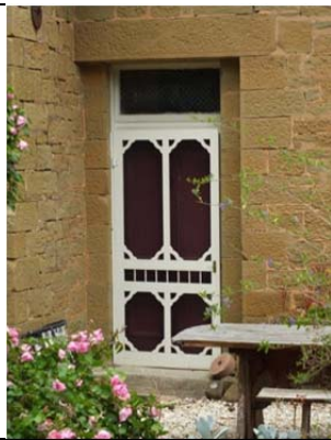
Photo 39: Former manse, front doorway detail, November 2014.
