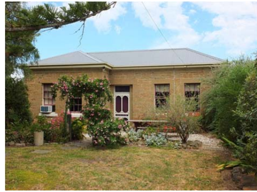
Photo 38: Former manse, north elevation, November 2014.
