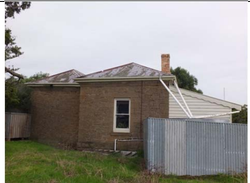
Photo 42: Former manse, west elevation, April 2014.
