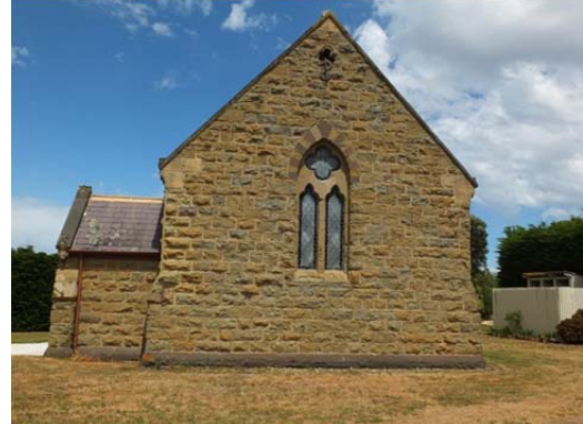
Photo 14: Barrabool Uniting Church, north elevation, November 2014.
