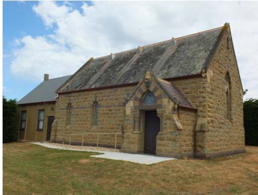
Photo 9: Barrabool Uniting Church, east and north elevations, November 2014.
