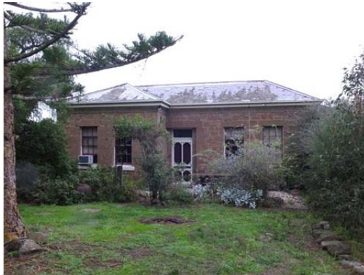
Photo 37: Former manse, north elevation, April 2014.
