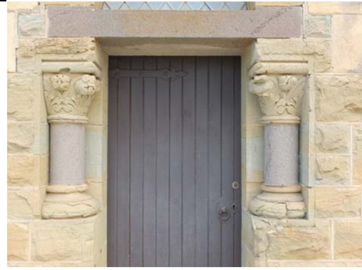
Photo 12: Barrabool Uniting Church, porch entrance detail (east elevation), November 2014.
