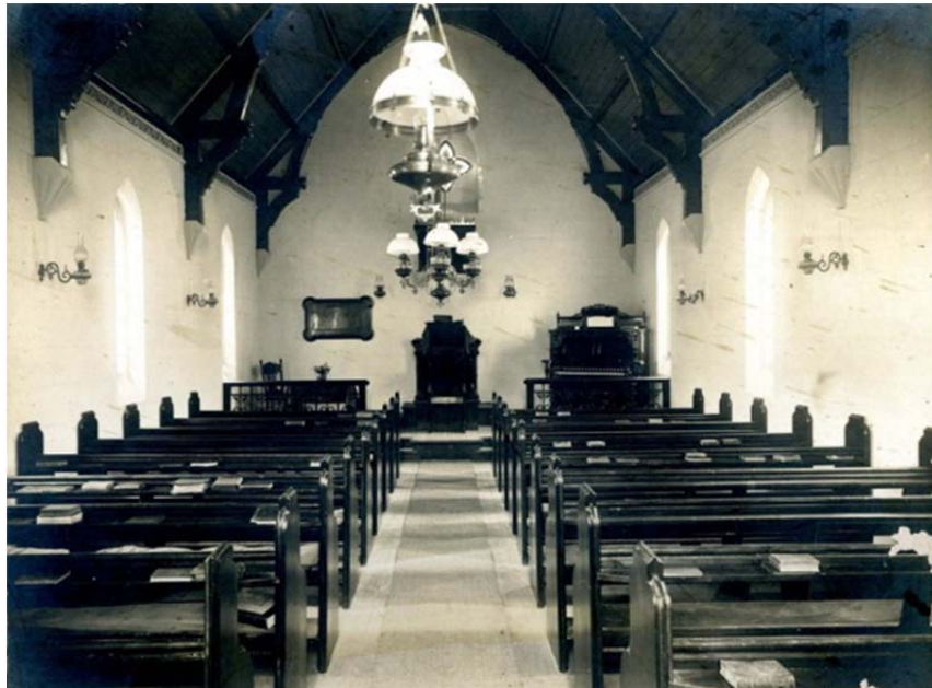
Figure 10: Barrabool Presbyterian Church looking south to pulpit, 1909.
