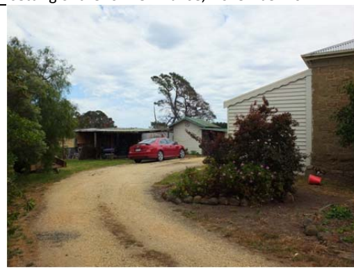
Photo 8: Gravel driveway to east of former manse and rear outbuildings, November 2014.
