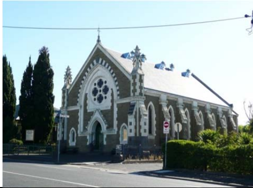
Figure 15: Former Newtown Free Methodist Church. Source: Victorian Heritage Database online.
