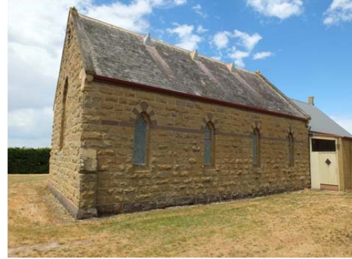
Photo 13: Barrabool Uniting Church, west elevation, November 2014.
