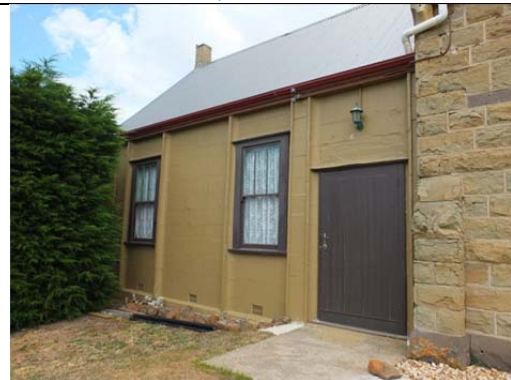
Photo 16: Sunday School Room addition, east elevation, November 2014.
