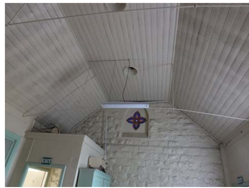
Photo 34: Sunday School Room interior, ceiling detail, November 2014.
