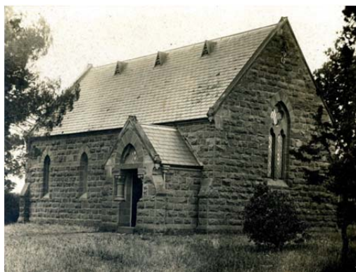
Figure 7: Barrabool Presbyterian Church, n.d. [1909]. Source: Adrian Schonfelder, National Trust of Australia (Victoria), Geelong & Region Branch.
