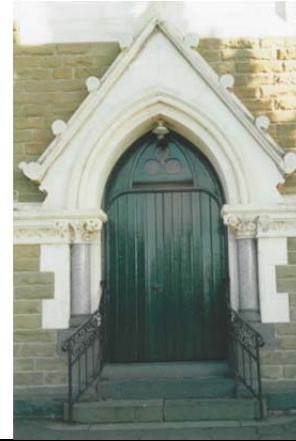
Figure 16: Detail of main doorway with squat piers with foliated capitals, 1991. Source: David Rowe.
