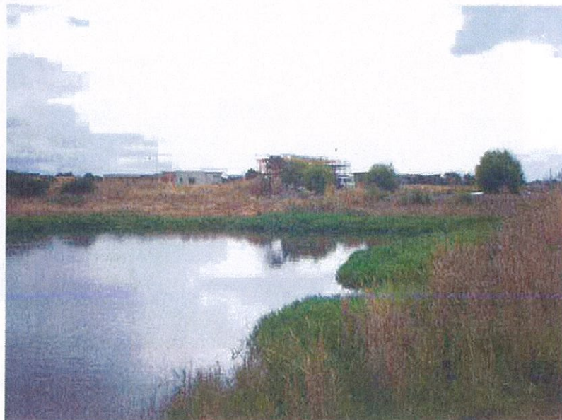
Figure 2 - Existing Detention Basin
