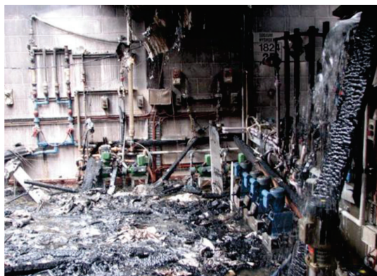
Figures 24 and 25: Damage to a water pumping plant which occurred during the 2009 Black Saturday fires
